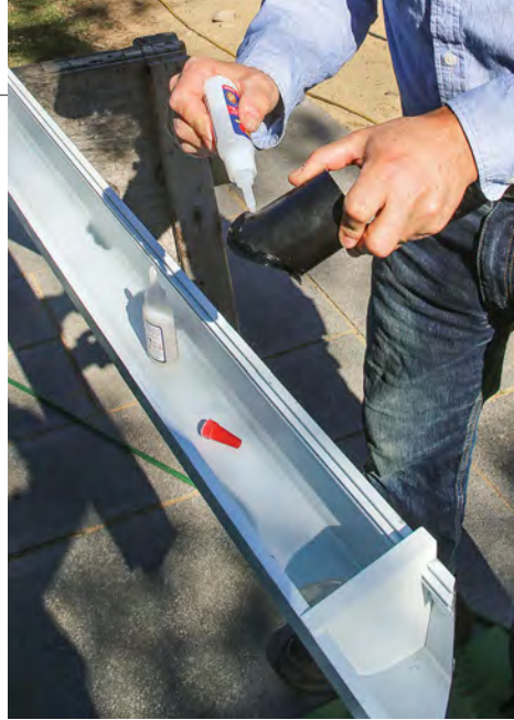
Glue the tube. CA glue is placed around the flange at the top of the downspout outlet. The outlets are ABS plastic, which is durable in warm and cold temperatures and UV-stable.
