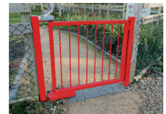
APSSTOP SHOWN IN GATE
