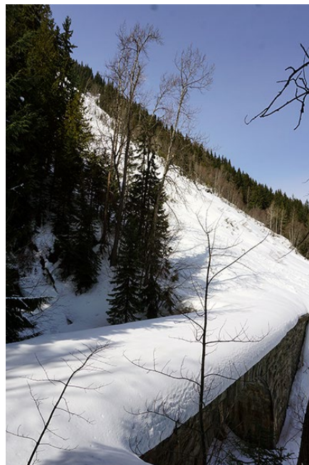
WP 10, Stone Arch bridge.
