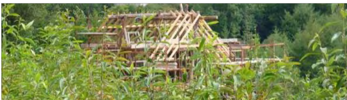
Pentiddy Woods, Cornwall: Acres of new chestnut and hazel coppice have been planted. The new house at Pentiddy is well screened by the existing and new hedges and woodland, and is constructed of locally sourced timber, milled on site, Delabole slate and Bodmin granite.
