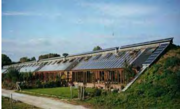
Hockerton Housing Earth-sheltered terrace
