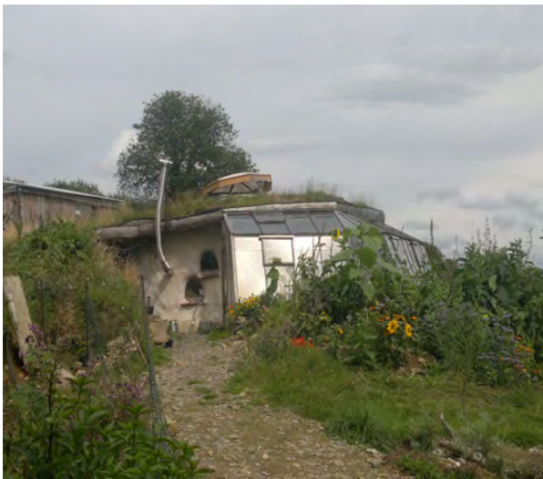
House at Lammas entirely powered by renewable energy. Photovoltaics power lights and computers and timber from the site is harvested, stored and used for cooking and to heat living space and water.
