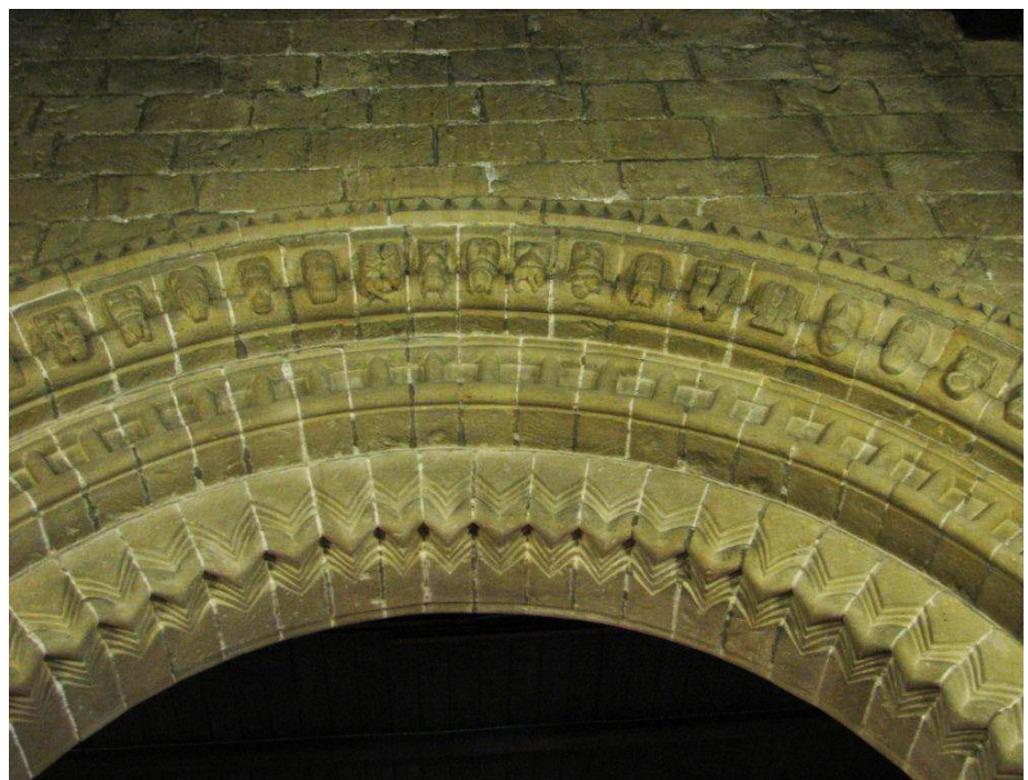
Photo 2. Beakheads on the chancel arch, St. John the Baptist, Adel, UK. Photograph, author.
