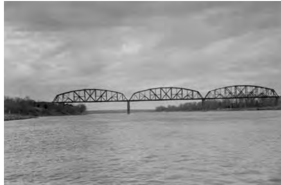
Bismarck-Mandan Rail Bridge, April 2023. HAER ND-2-10
