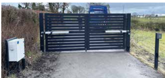
▲ Swing gates with above ground automation
