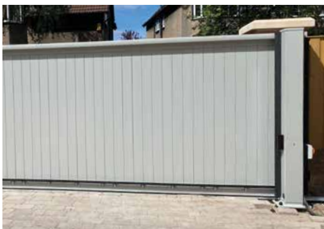
▲ Inside view of the gate showing the track
