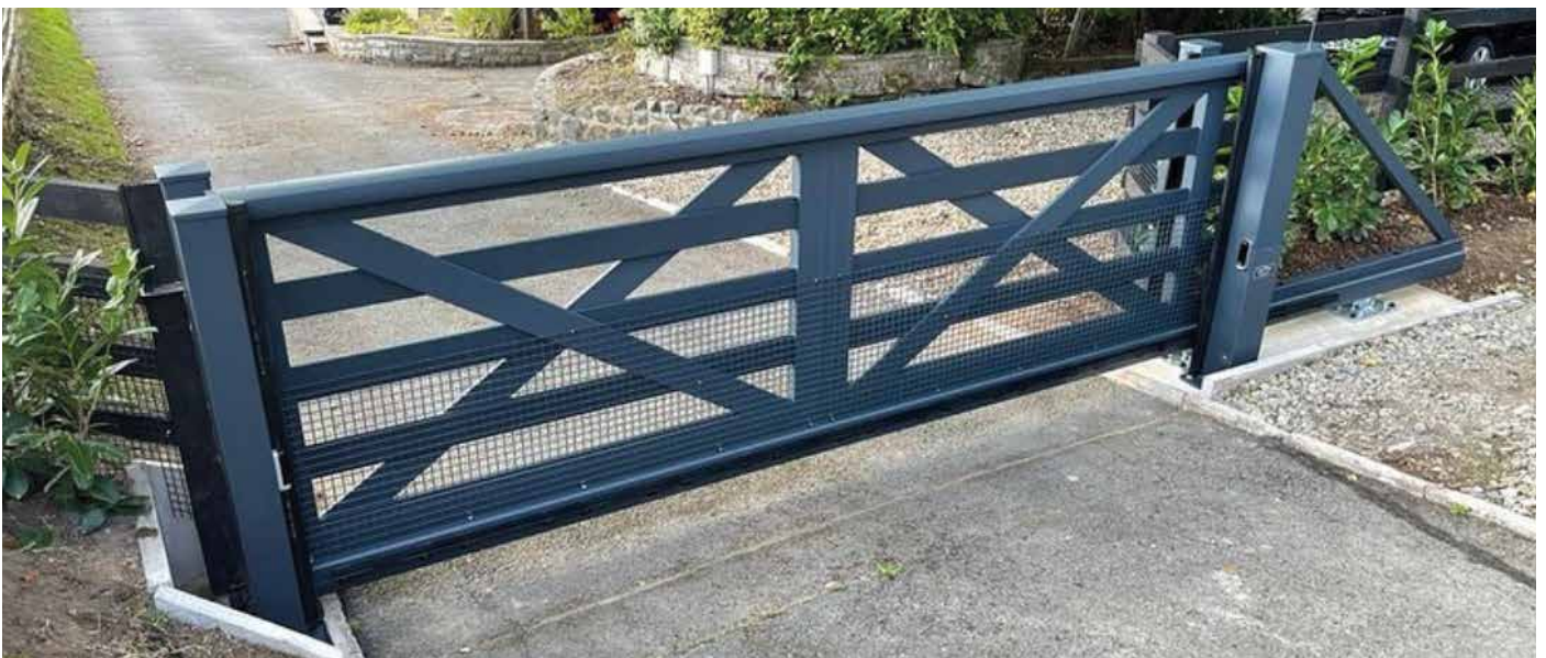
▲ A traditional five barred design made into a sliding gate
