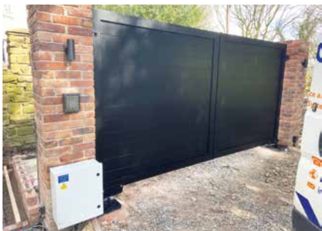
▲ Swing gates with underground operators
