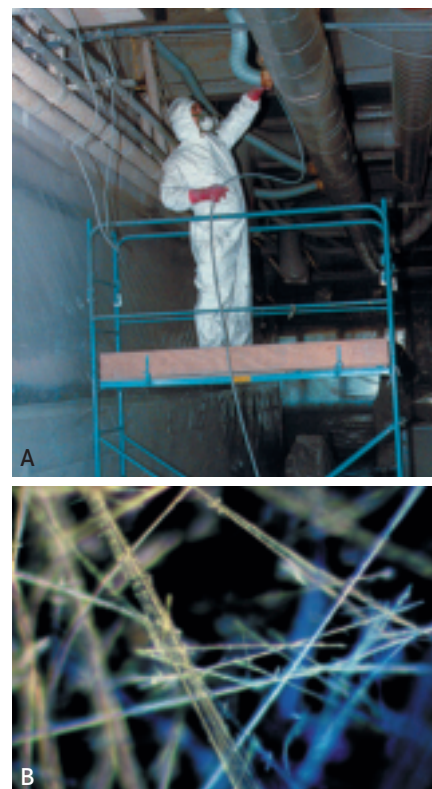
Fig. 2.17 Asbestos insulation is common in buildings and presents a hazard when disturbed during demolition. (A) Protective clothing must be worn to avoid contact with (B) asbestos fibres .
