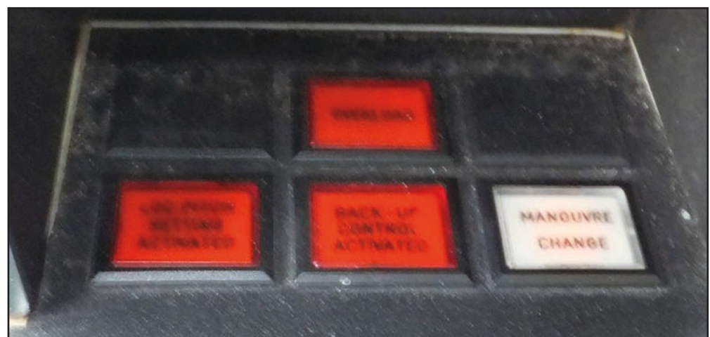
Figure 2: Bridge wing console CPP back-up control system indicator lamps
