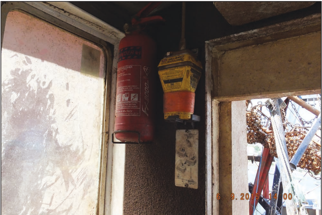
Figure 31: JMT 's EPIRB located on the wheelhouse bulkhead
