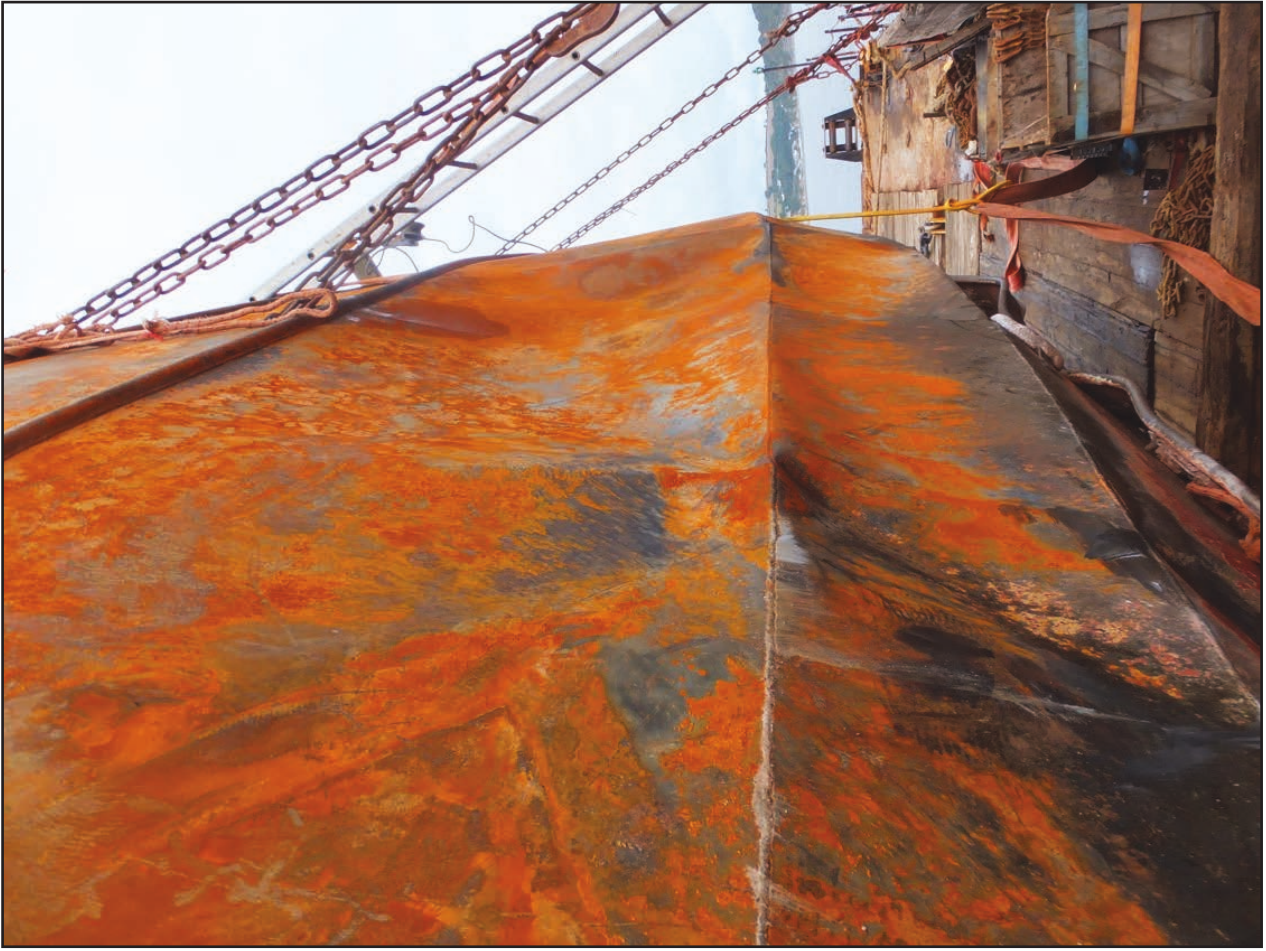
Figure 27: Implosion damage to JMT's port side
