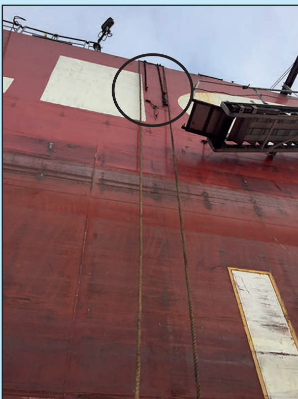
Figure 2: Ladder rigged position, showing broken section
