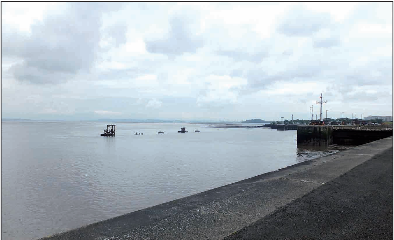
Figure 1: View of exposed dolphins
