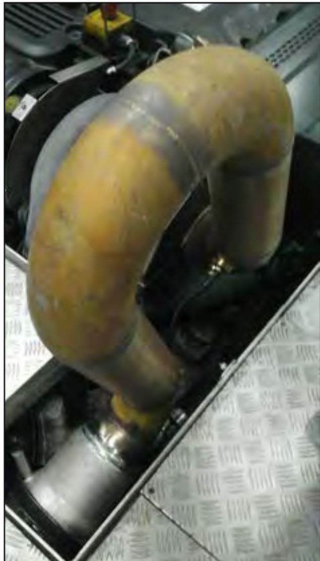
Figure: Starboard engine exposed exhaust pipe
