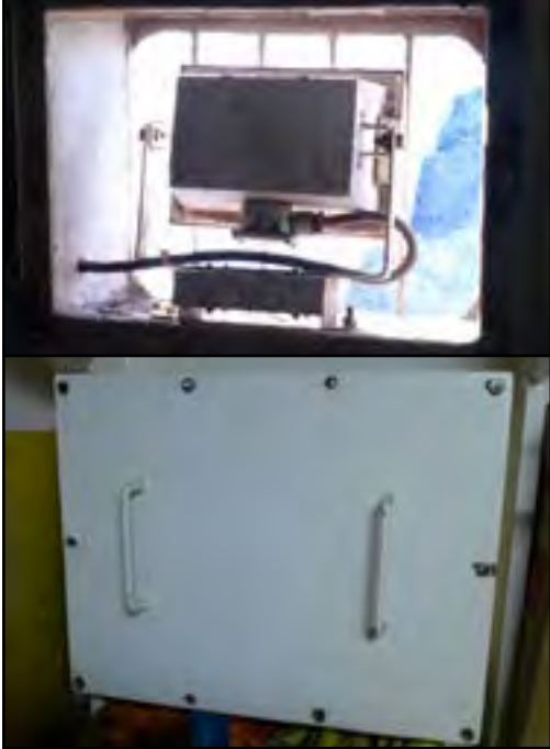
Cargo lamp access plate (removed and closed)
