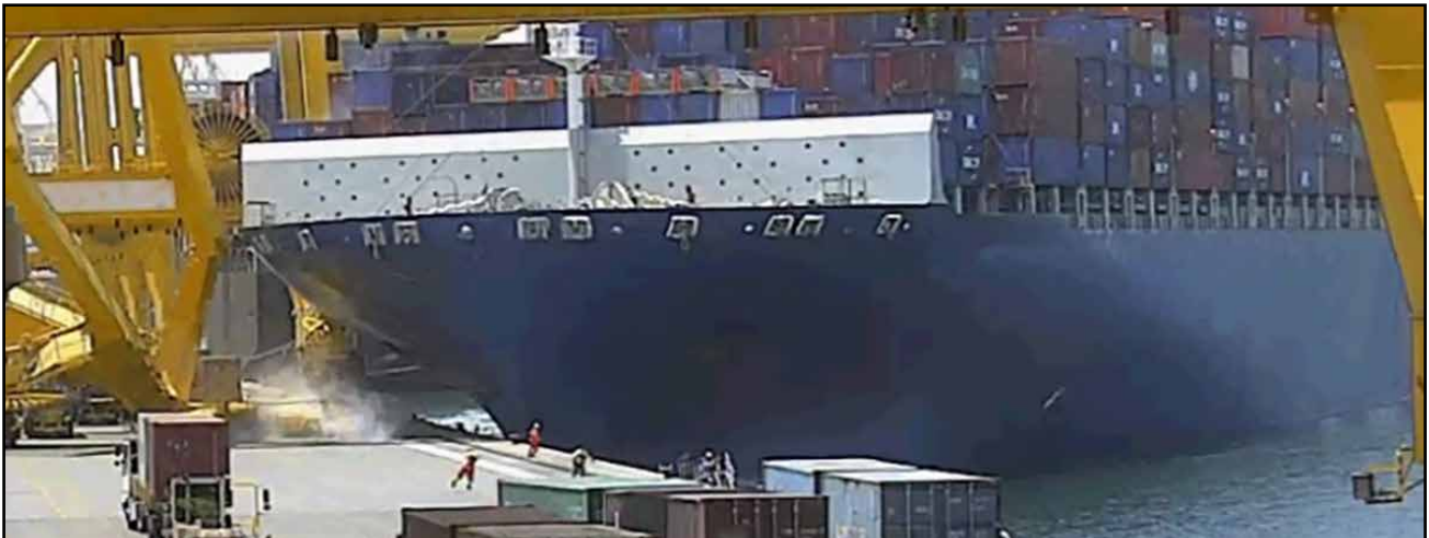
Figure: The container ship's bow making contact with a crane
