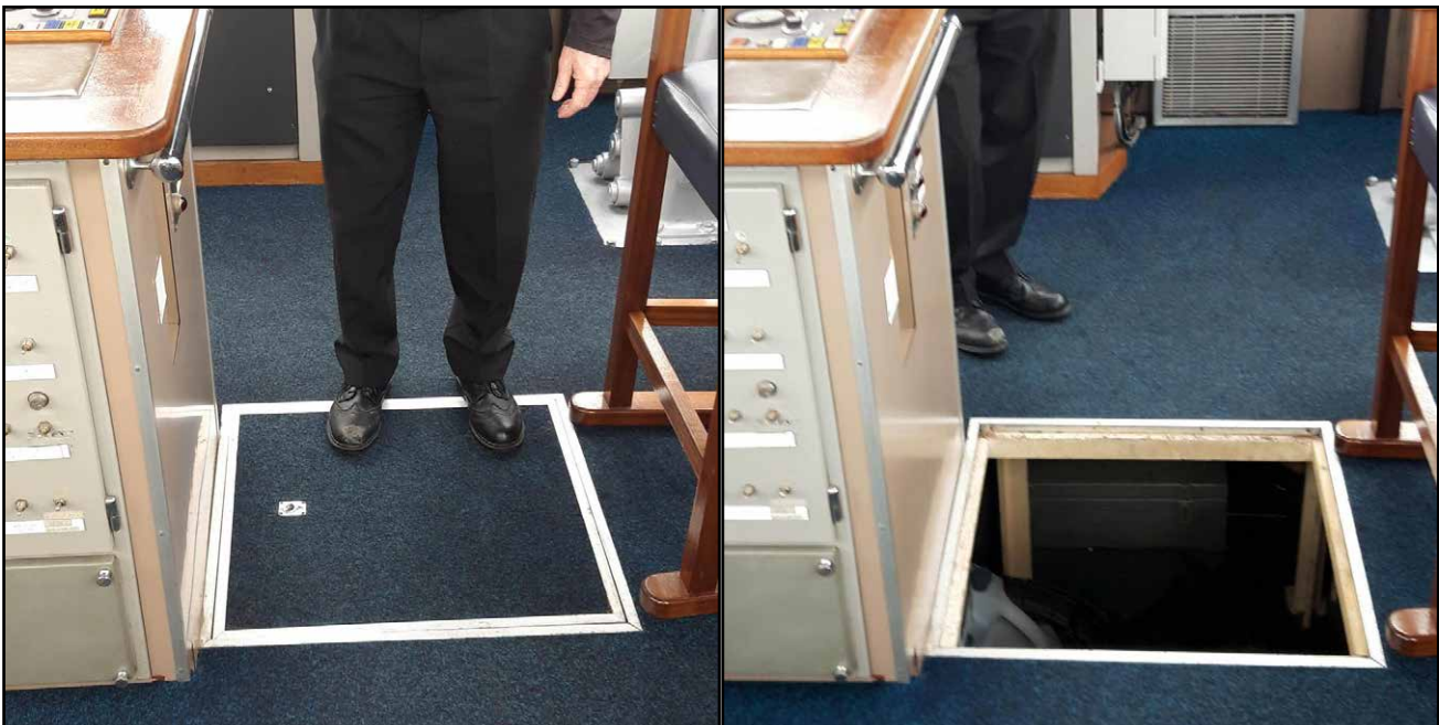
Figure: The wheelhouse access hatch shut and access hatch open
