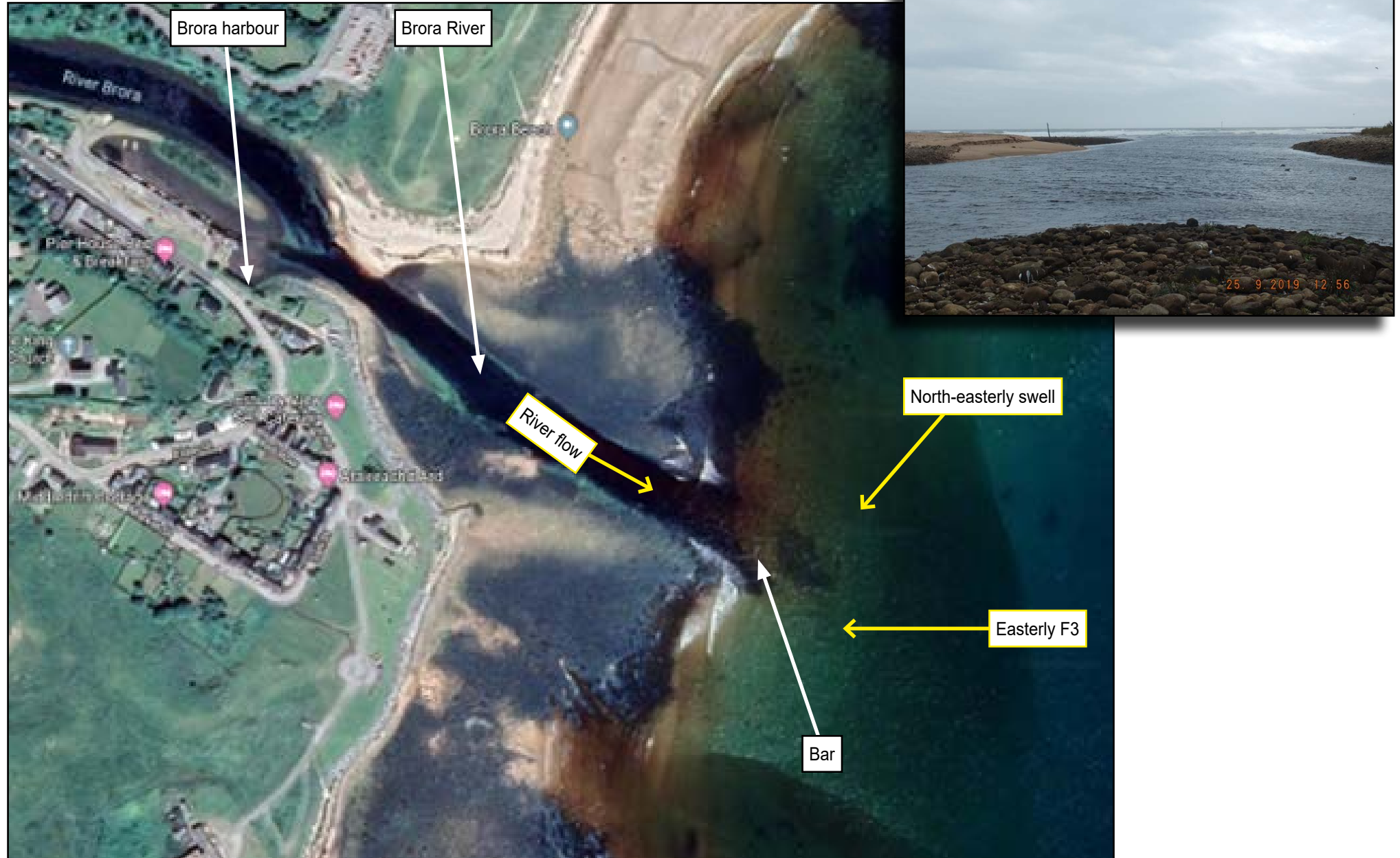
Figure 2: Satellite image of Brora river entrance (inset: looking from Brora harbour towards the river entrance)
