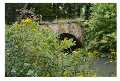
The sidewalls have wide, flat capstones with rusticated faces. The bridge deck is covered with asphalt between the sidewalls. The Franklin Street Stone Arch Bridge is one of four large single-arch stone bridges in Carroll County. Three of these four were constructed by local mason, John C. O'Connor, in the early 1900s, including the Franklin Street span. The bridge embodies the importance bridges served to the early development of
