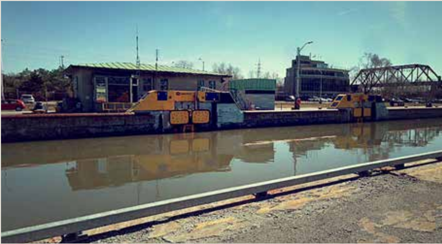
The Saint Lawrence lock equipped with suction cups.
