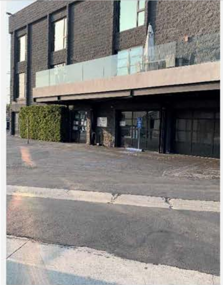
3: External Photo Facility Building
