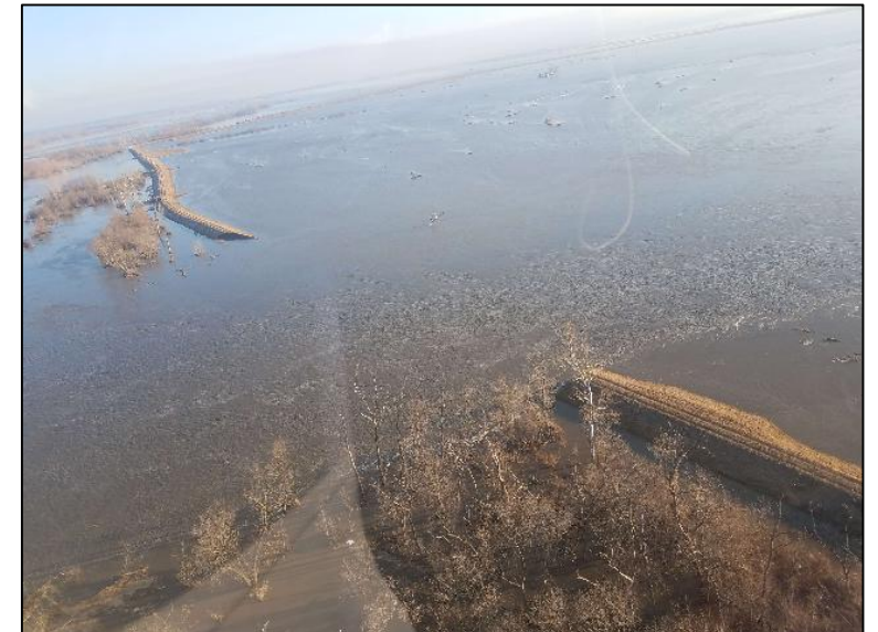
L-575 levee breach along the Missouri River near Percival, IA impacted I-29 (2019)
