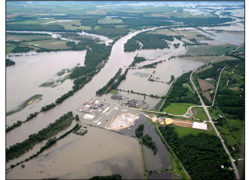
Missouri River flooding near Fort Calhoun nuclear plant, Blair, NE (2011)
