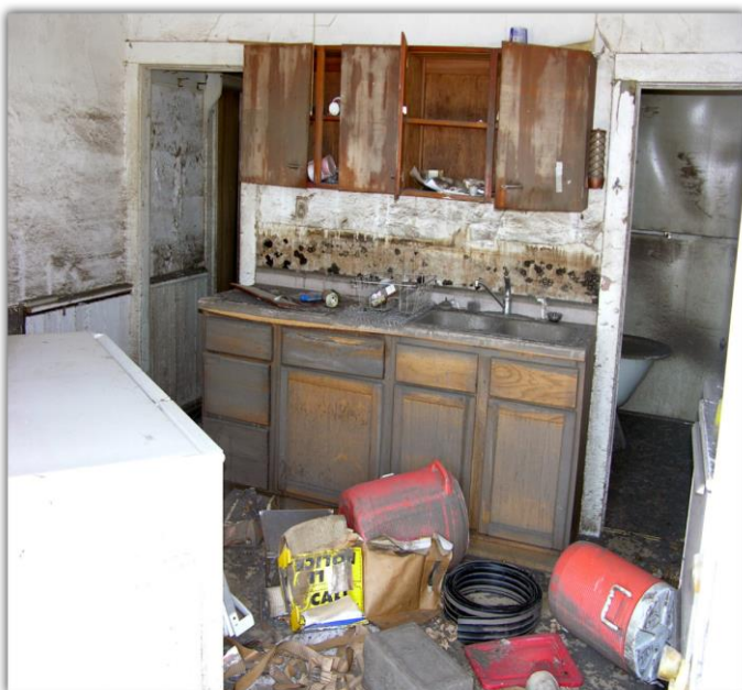
Figure 8. A Cedar Rapids home damaged by the 2008 flood.
