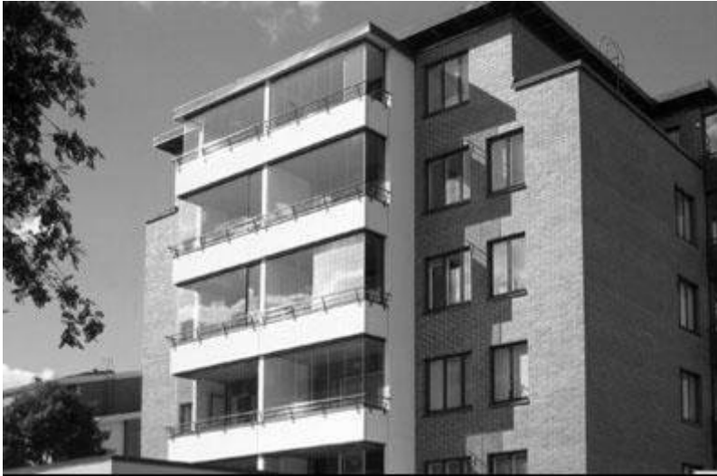
Figure 1. Balconies made of reinforced concrete and outfitted with glazing.
