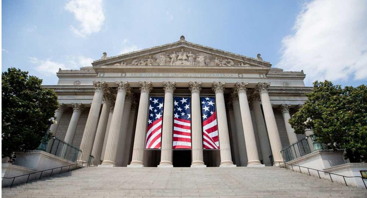
The National Archives Building, designed by renowned architect John Russell Pope (1874-1937), Washington, D.C. (National Archives)
