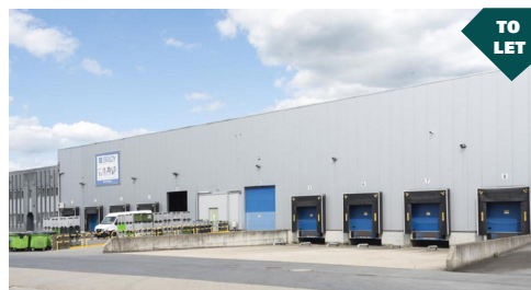
▶ ZELE ▶ Warehouse 12.300 sq m + Offices
