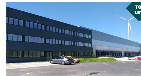
▶ BILZEN ▶ Warehouse 19.985 sq m + Offices
