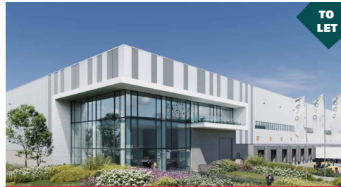
▶ GRIMBERGEN ▶ Warehouse 21.238 + 31.416 sq m + Offices
