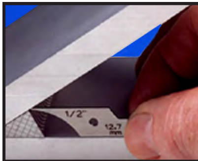
CHECKING WELD DIMENSION OF SKEWED MEMBER
