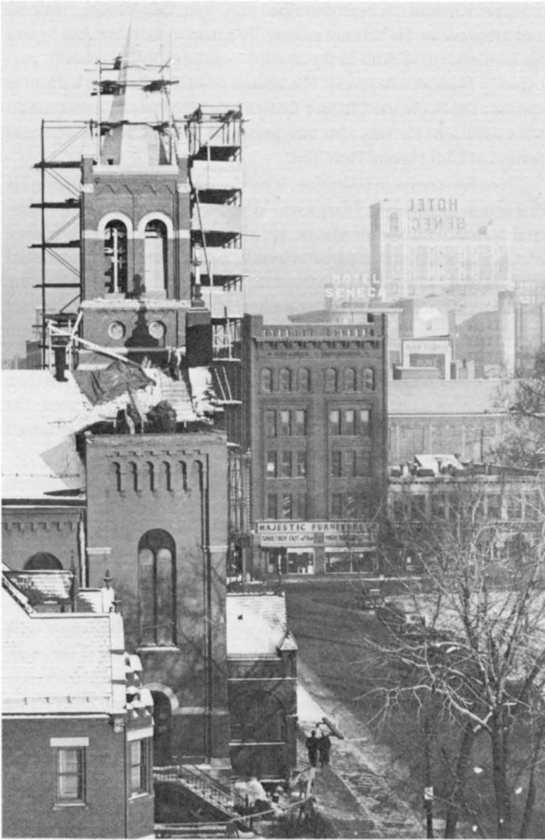
Construction of St. Mary's Church Belfry, 1940
