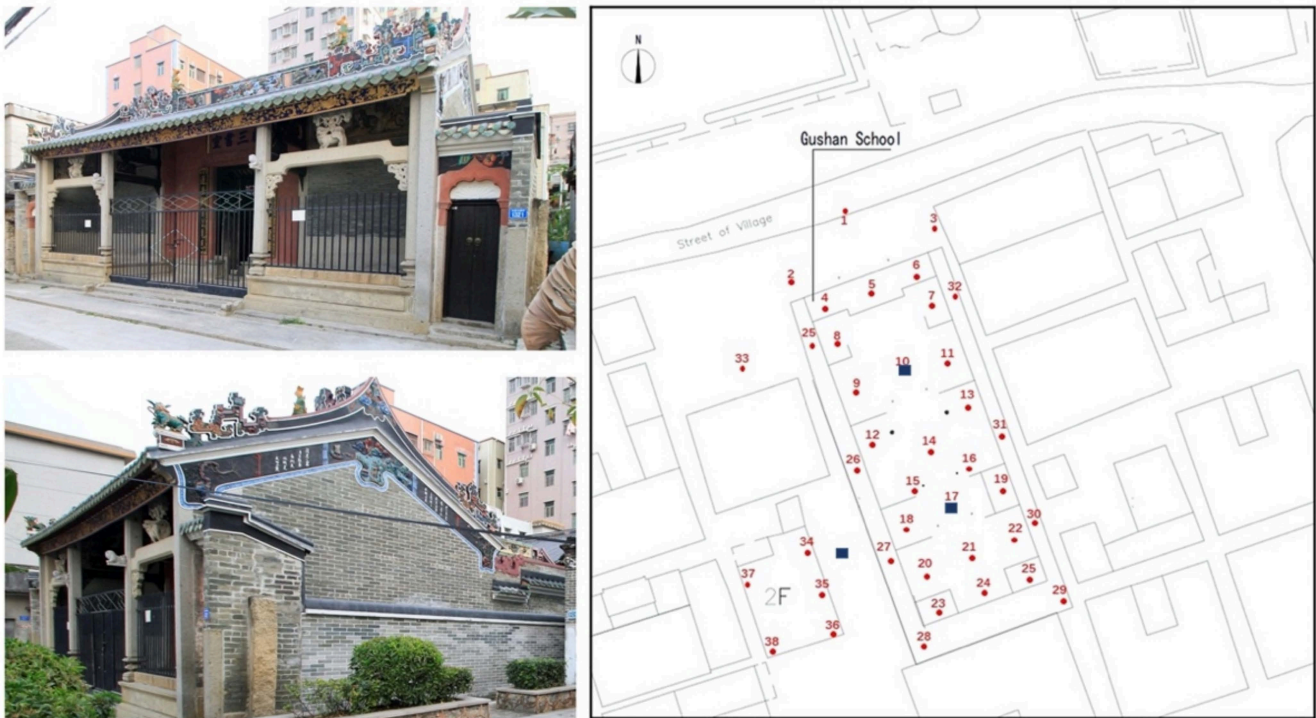
Figure 4. Outdoor scanning arrangement of the Gushan school. In all, there are 36 scanning stations arranged for the outdoor scanning of the Gushan school.
