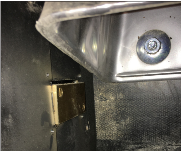
Rub-Block RB200DN view from inside the elevator.
