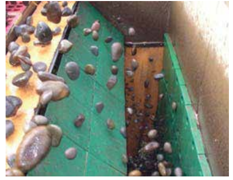
REDI-LINER™ solid urethane installed after screen overshoot area
