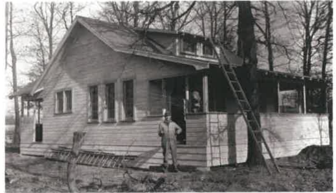
Lloyd and Gordon Ray building a cottage. Collections of the Dunn Museum.
