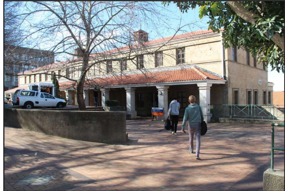
Image: Western approach, facing towards the building.
