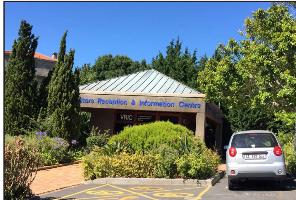
Image: Centre as seen from the vehicular approach.
