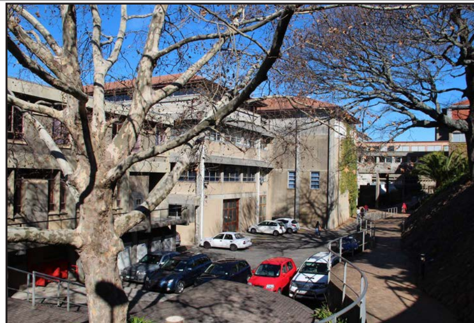
Image: Portion of the space between the Library, Menzies & west bounding retaining wall.
