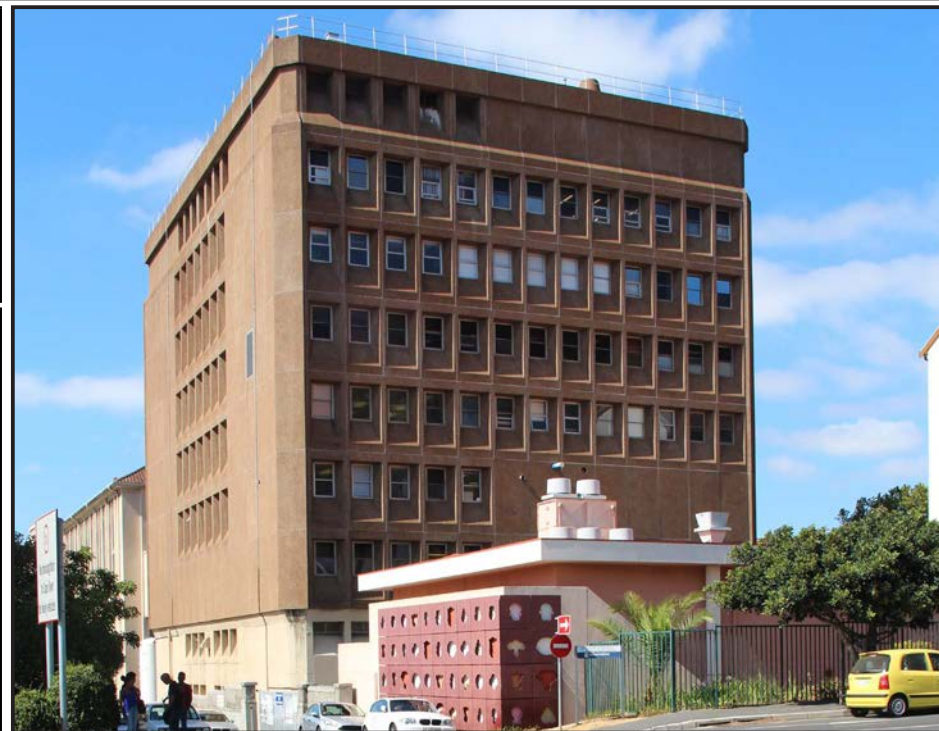
Image: View of the northern facade of the building, as seen from Anzio Road.
