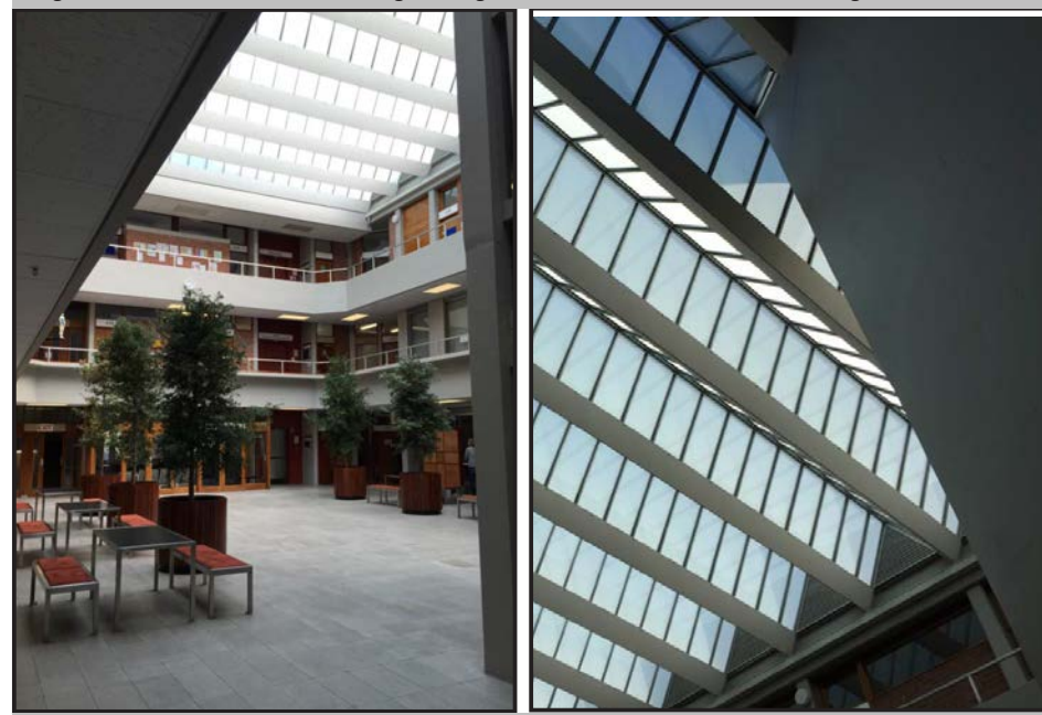
Image: Interior view of the central atrium (L); View of the glass saw tooth roof over the atrium (R).
