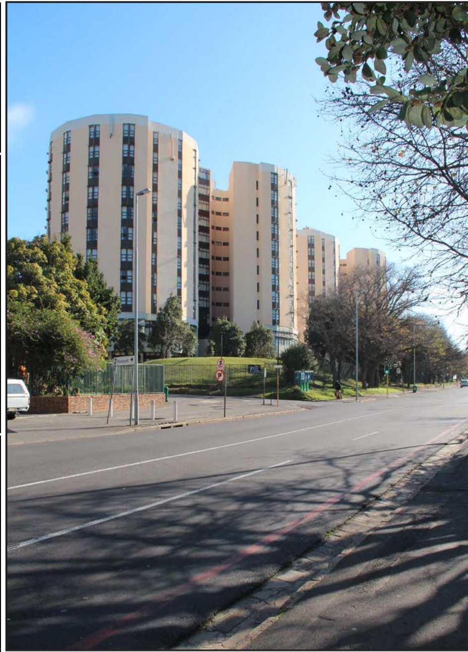
View across Main Road looking north towards the building.
