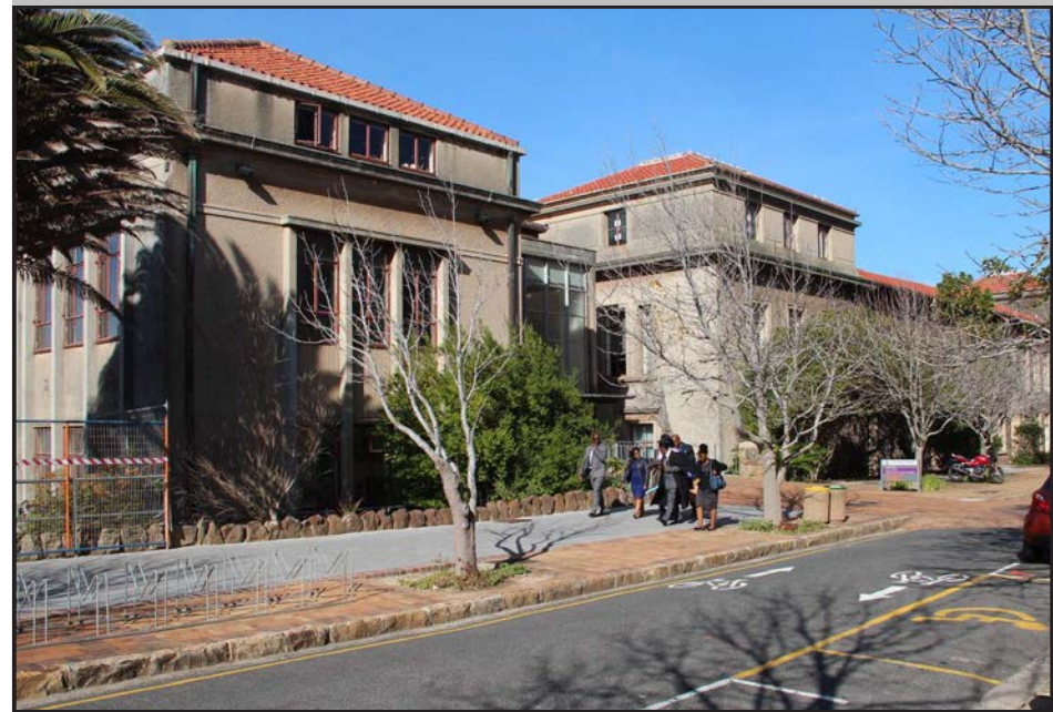
Image: View of the building from a northern approach.
