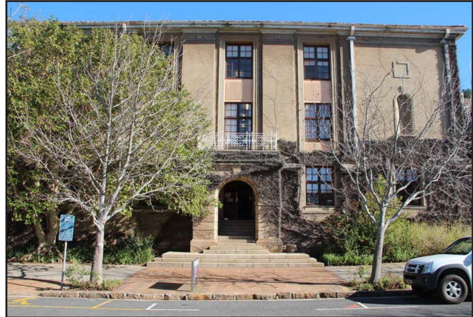
Image: East facade of the mid-20th Century section of building, as seen from University Avenue North.
