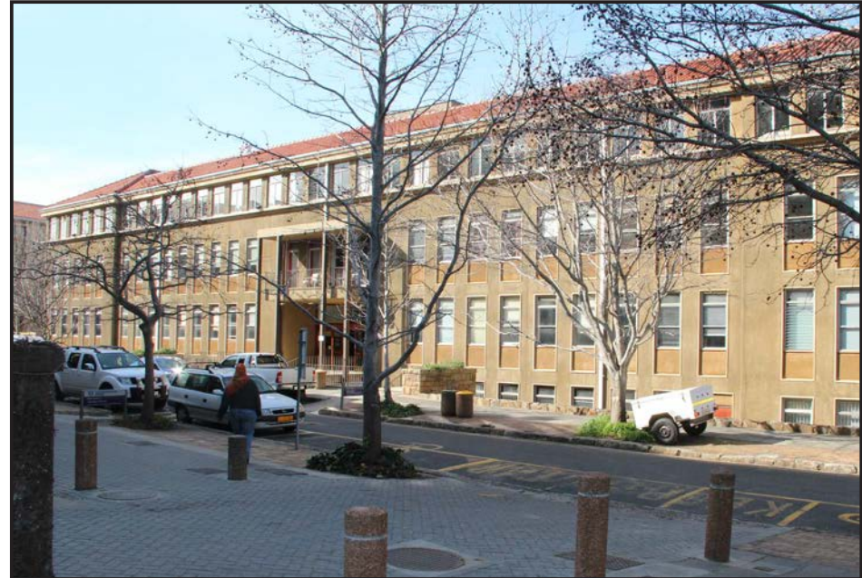
Image: View of the building as seen from University Avenue South.
