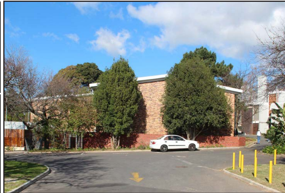
Image: View of the northern facade of the squash courts.
