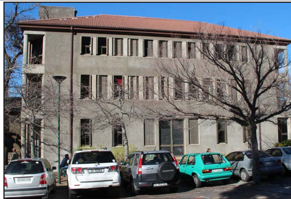
Image: West facade and entrance to the Oppenheimer Institute.
