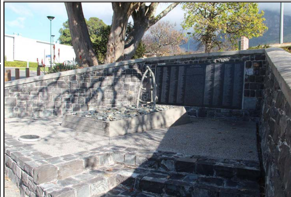
Image: View of the memorial, recently upgraded and restored by Thorold Architects.
