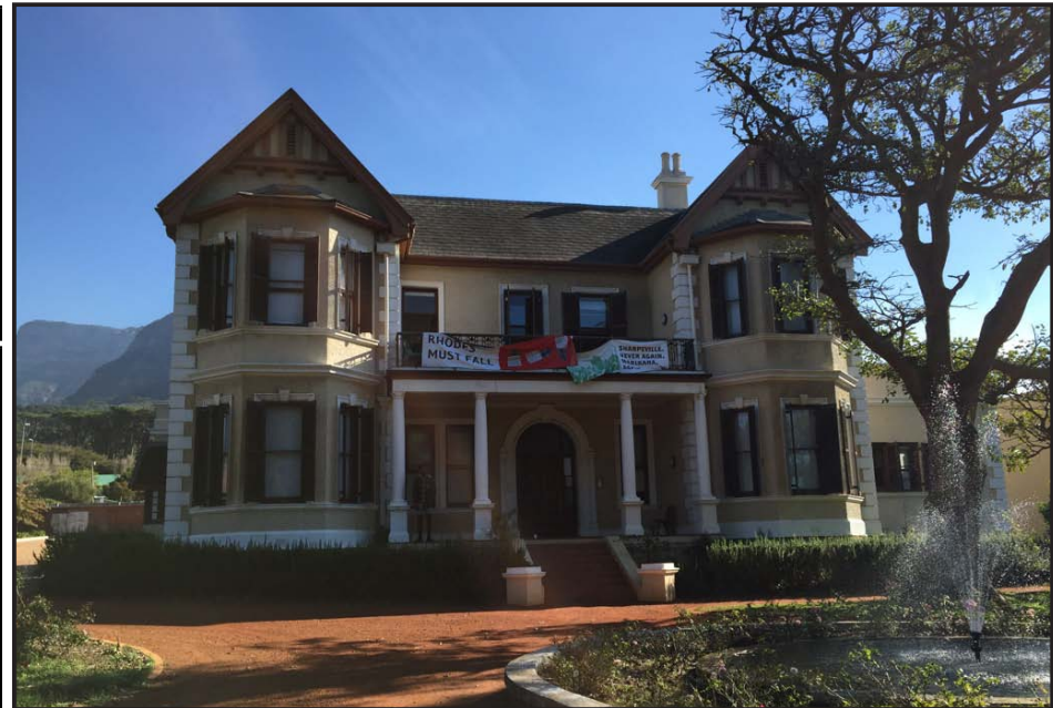
Image: View of the primary east-facing facade of the house.
