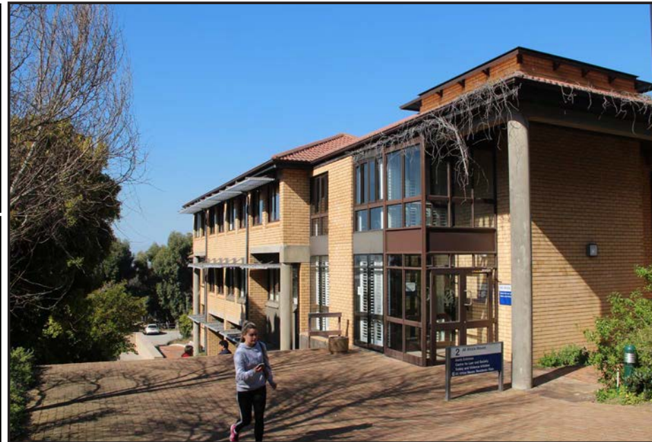
Image: Photograph looking east with a view of the northern facade of the building.
