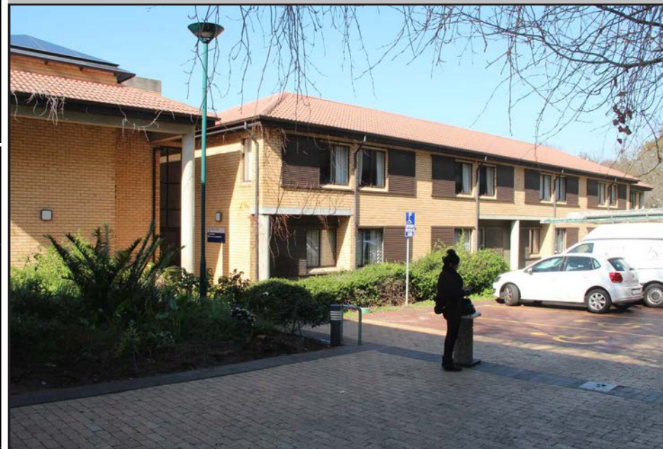
Image: View of the eastern facade of the building.
