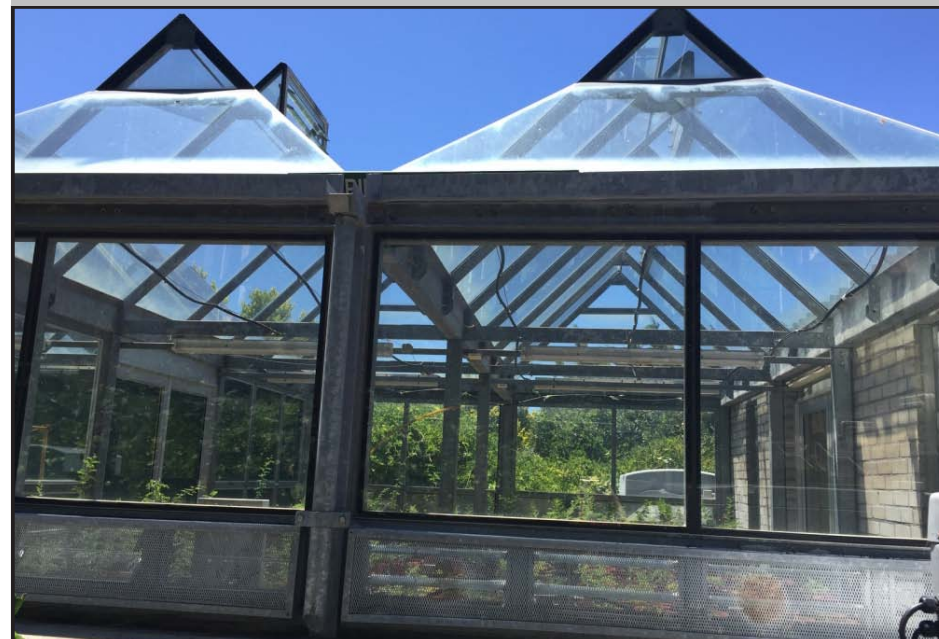
Image: Detail of a section of the glass house.
