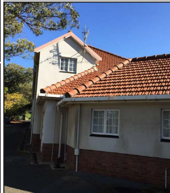
Image: View looking up along the south-eastern facade.
