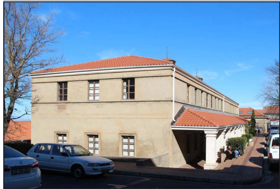
Image: North facade of the building.
