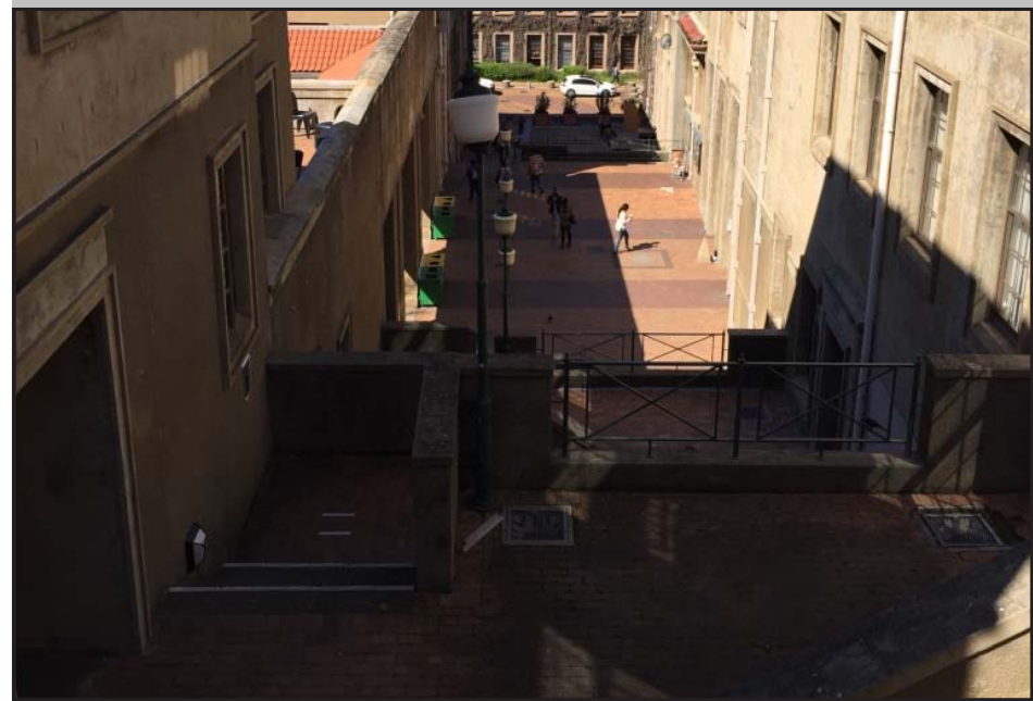
Image: View looking down the stairway from the upper level of the Steve Biko Building.
