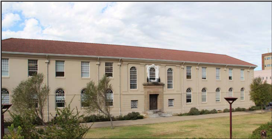
Image: View of the western facade.
