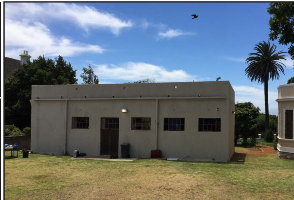
Image: View of the western facade of the building.
