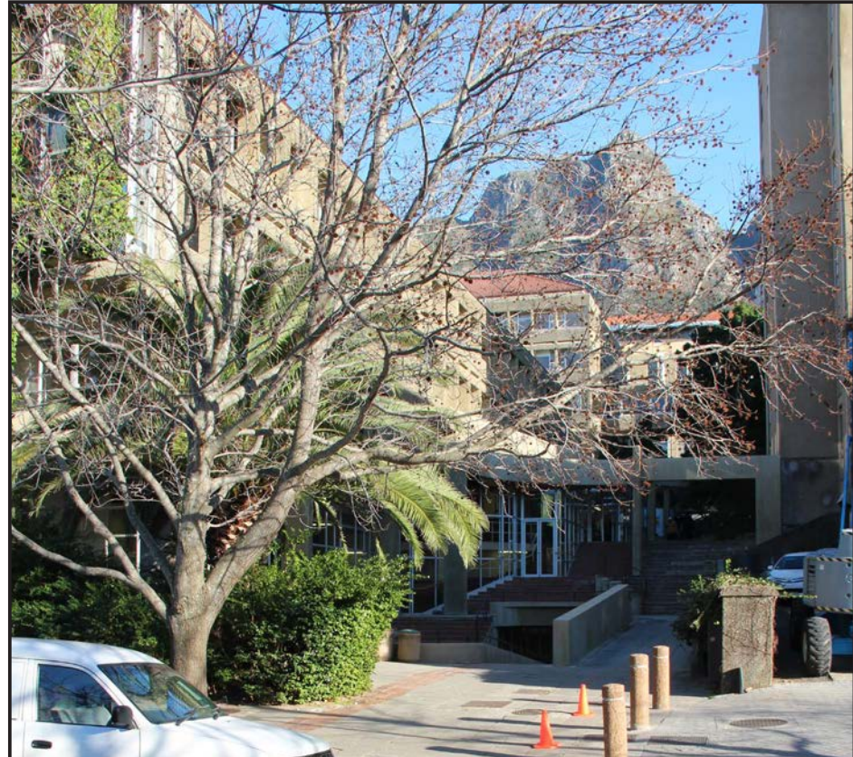
Image: View from University Avenue South toward the acces route.
