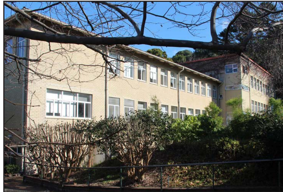
Image: North facade of the building.
