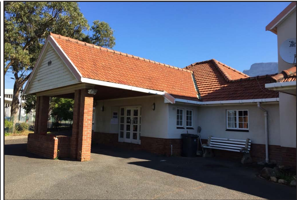
Image: View looking south towards one of the primary pedestrian entrances on the east facade.
