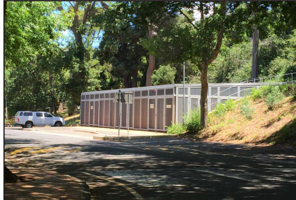
Image: View from Ring Road/Madiba Circle, approaching from the north.
