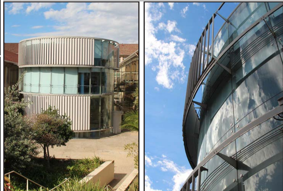
Image: View of the pavilion (L) and detail of the glass and shutter system (R).
