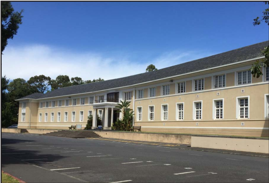
Image: View of the east-facing, primary facade and entrance to the building.
