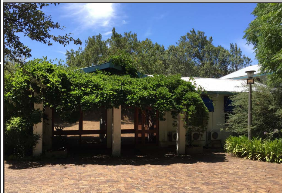
Image: View of the west facade of the building.
