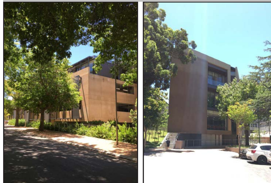
Image: Different exterior views of the New Snape Building.
