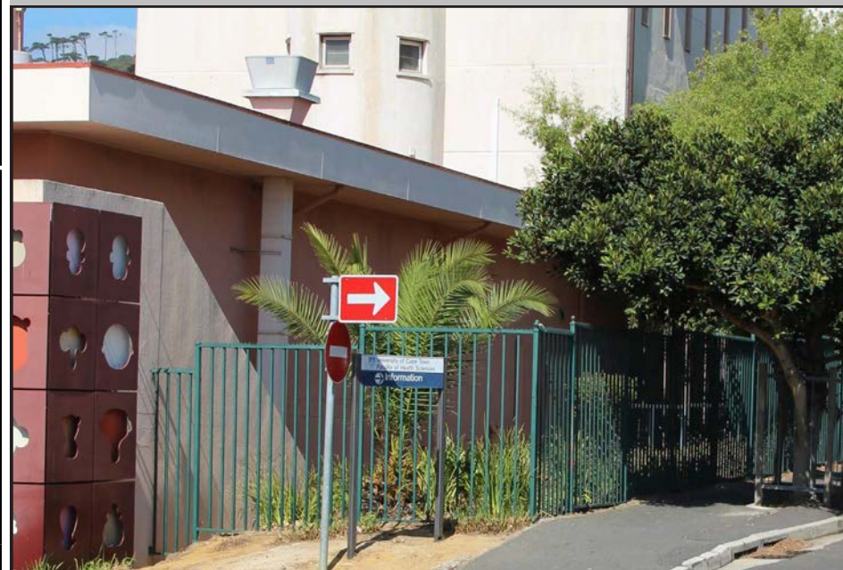
Image: Northern elevation of the Animal House along Anzio Road.
