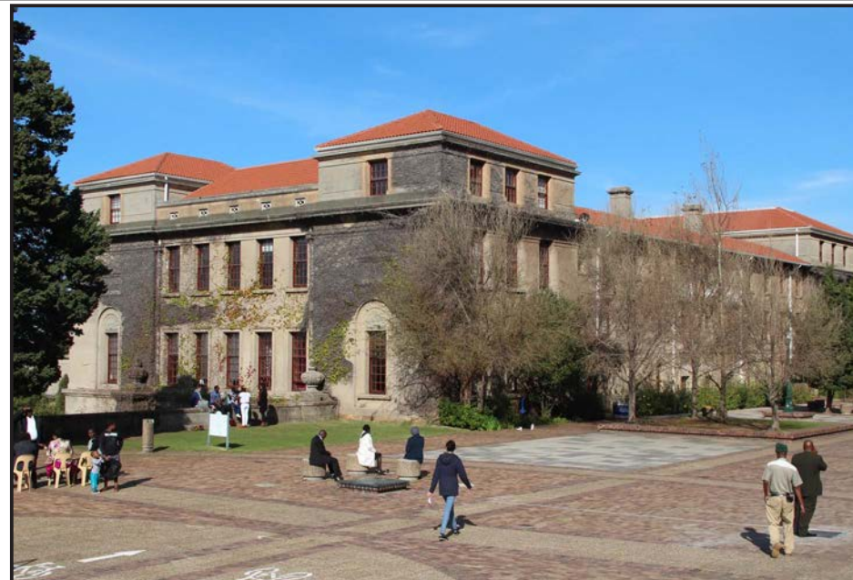
Image: View from Jammie Plaza toward the AC Jordan Building/Arts Block.
