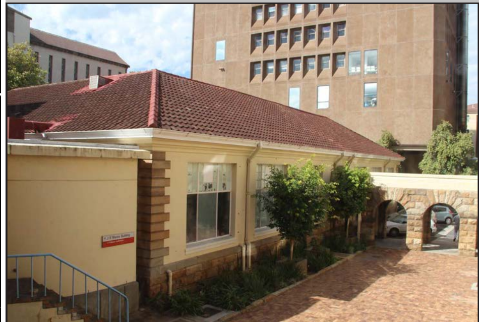
Image: Southern elevation of the mortuary, showing the bridge link to Wernher-Beit North.
