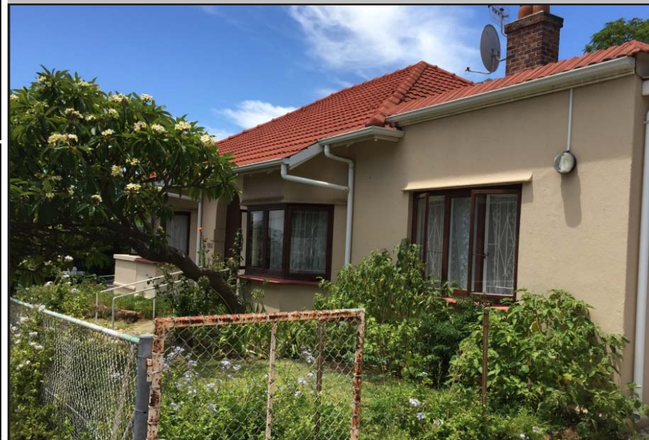
Image: View, looking east, of the northern facade of the house.
