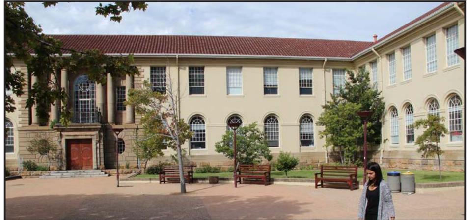
Image: Detail of the western facade of the building.
