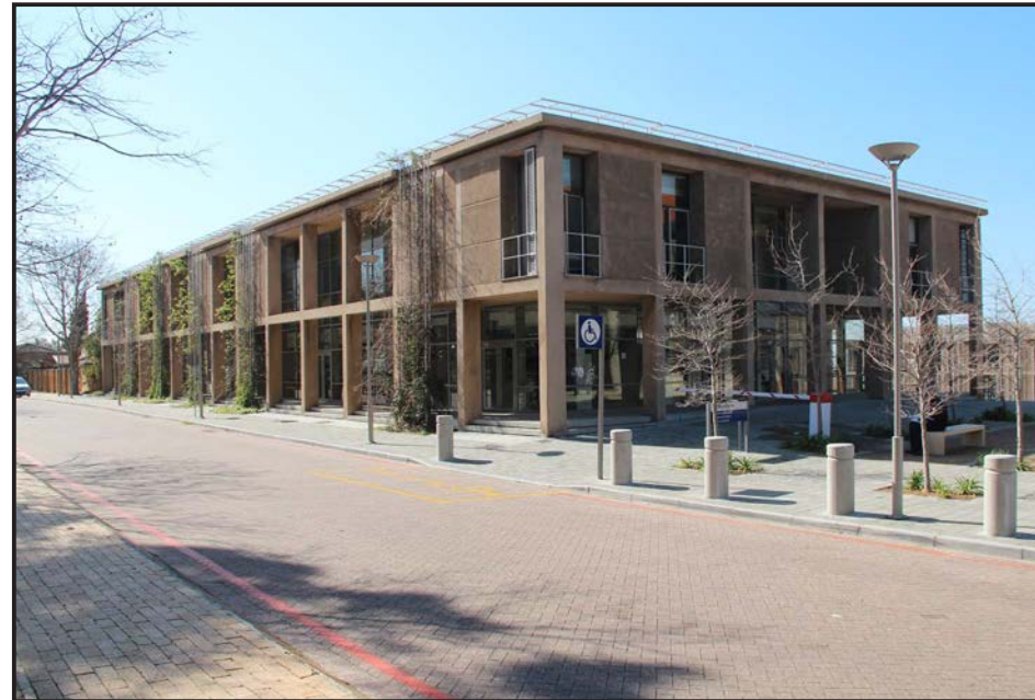
Image: The building as seen from the main vehicular thoroughfare through Middle Campus.
