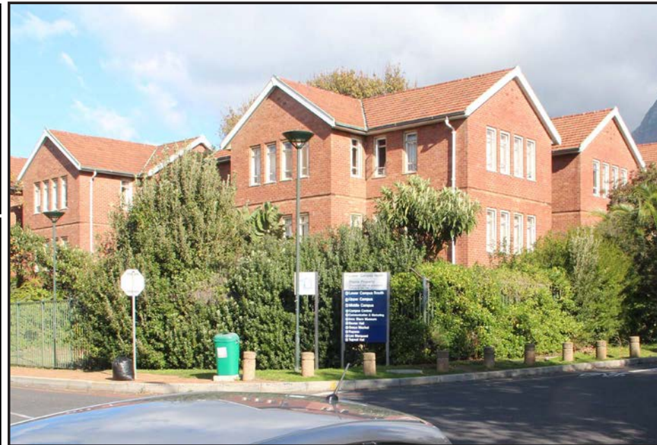
Image: View across the interchange between Chapel & Baxter Roads looking towards the building.
