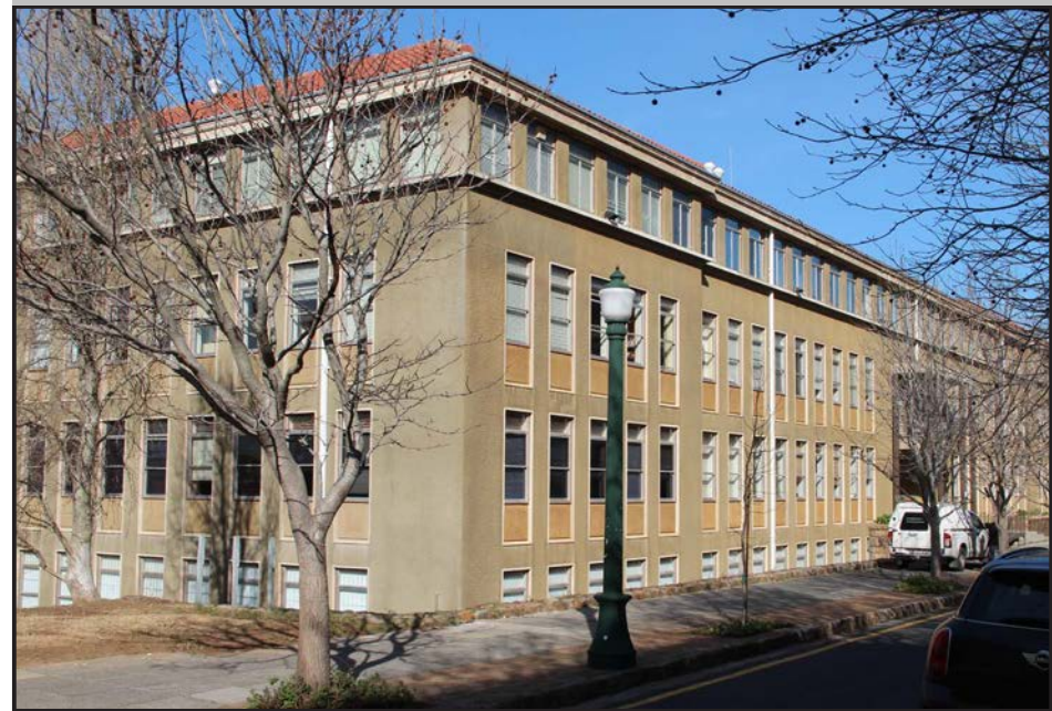
Image: Another view of the building from University Avenue South.
