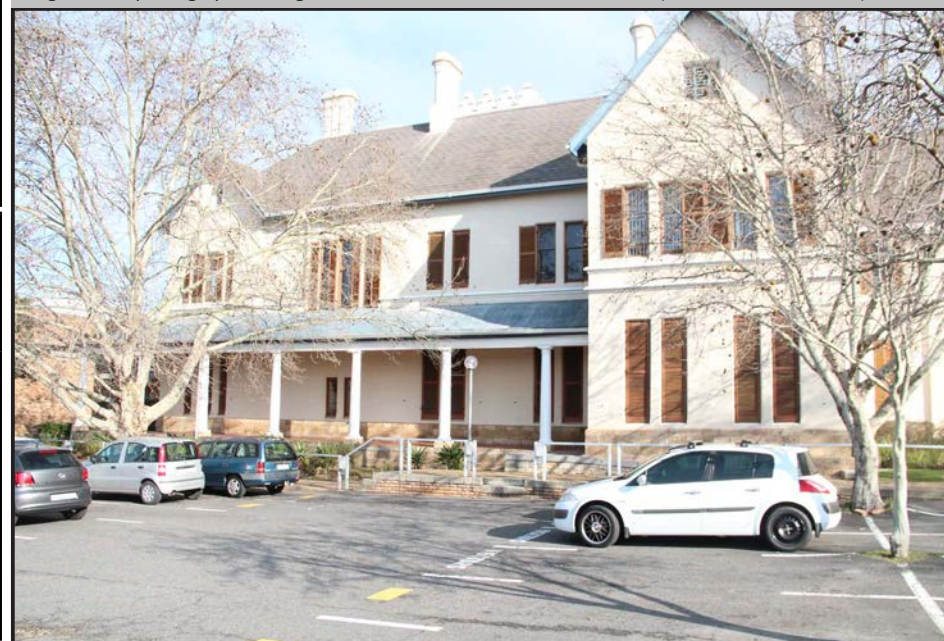
Image: View of the north facade of the building.
