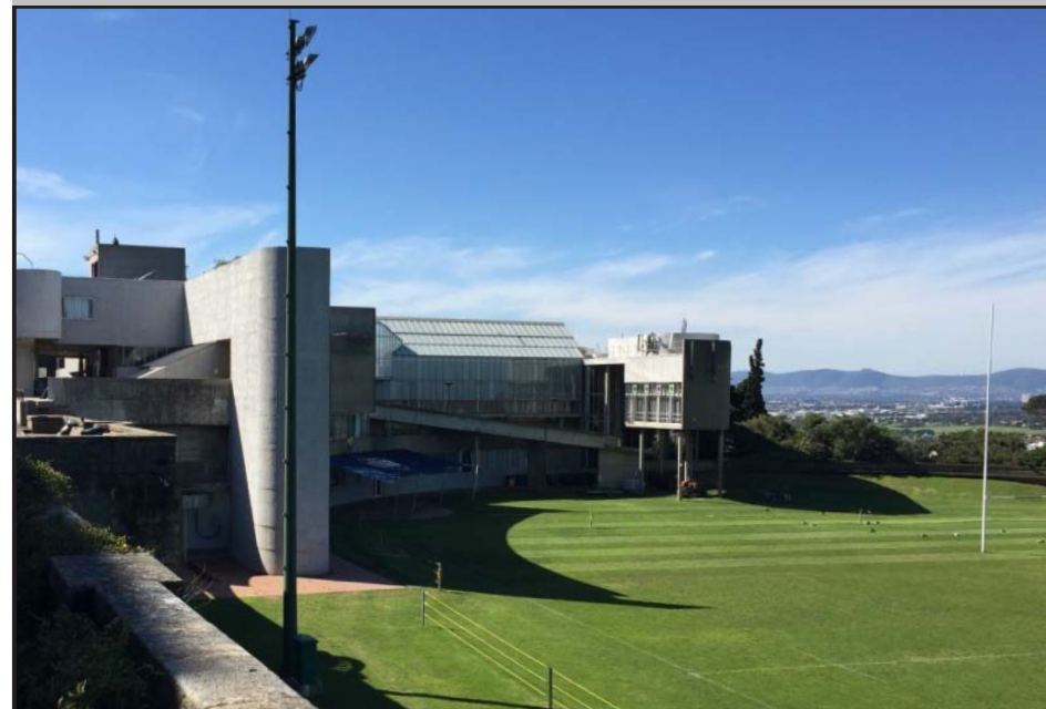
Image: View looking northwards from Rugby Road.
