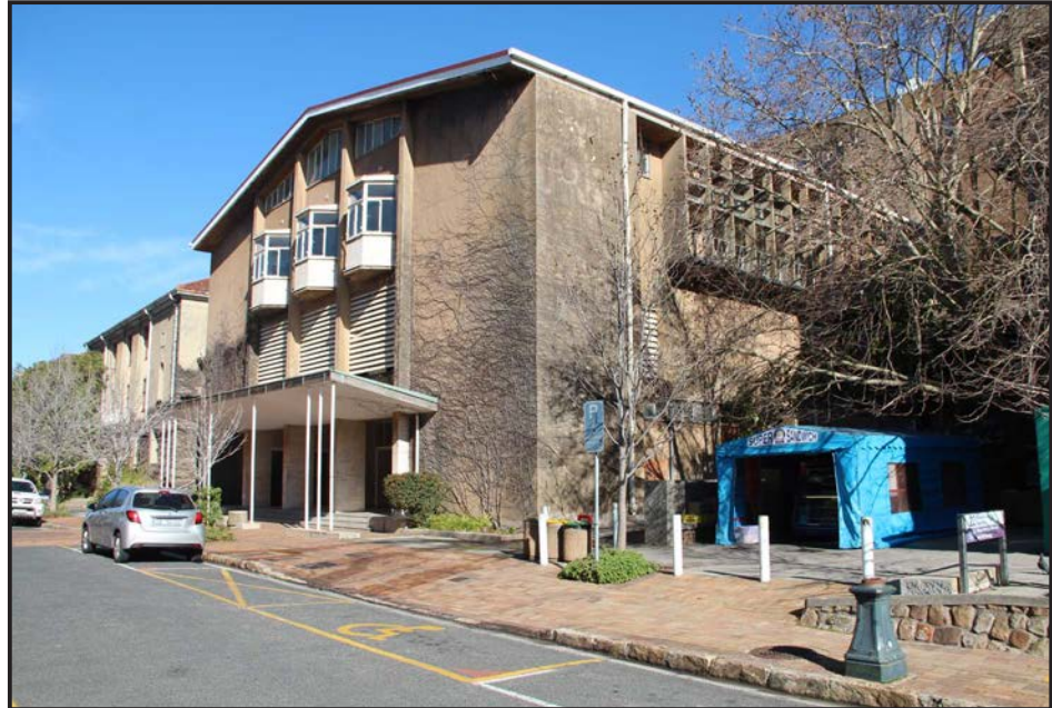
Image: View of the building from the north as seen along University Avenue.
