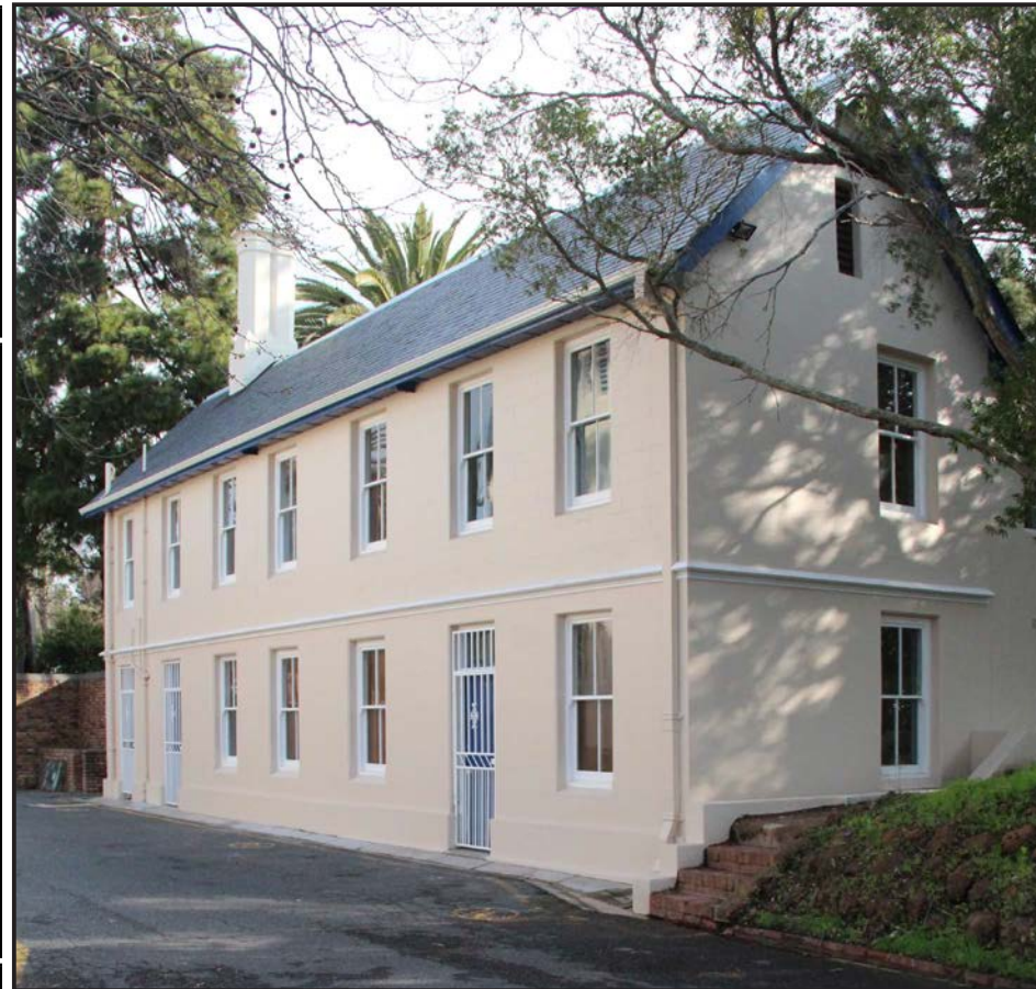
Image: View of the primary east-facing facade of the cottage.
