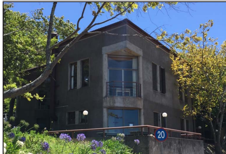
Image: View from Ring Road towards the south-eastern corner of the building.
