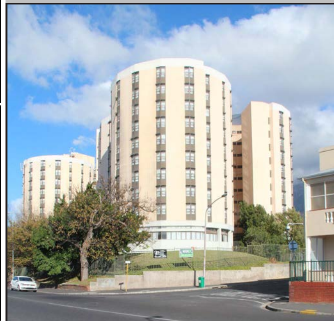
Image: View across Main Road looking south-west towards the building.
