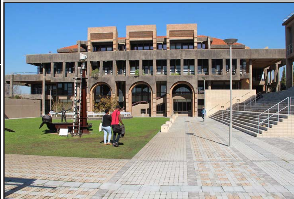
Image: Northern elevation of Kramer.
