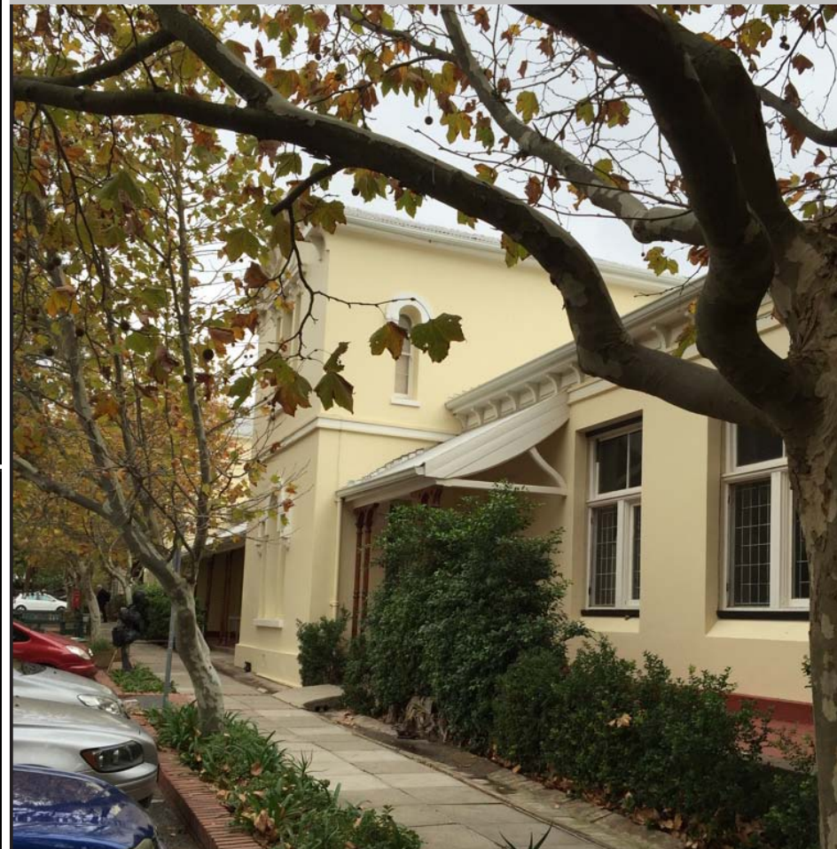
Image: View along the primary, east-facing elevation.
