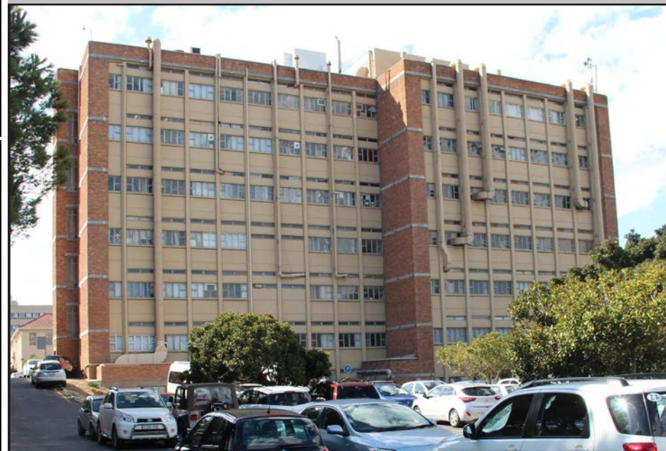
Image: The southern elevation of the building.
