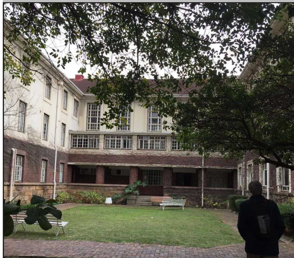
Image: View of the courtyard in the Medical Residence.
