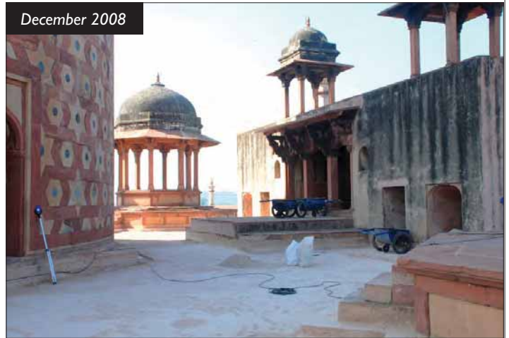
(Top) Over a million kilos of concrete laid since the 1920's has been removed from the roof.
