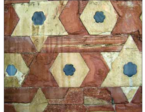
Almost 15% of sandstone on the neck of the dome is to be replaced
