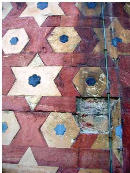
17 aluminium strips are presently installed in a rather intrusive and damaging manner. These will be replaced with a single system using copper cables.
