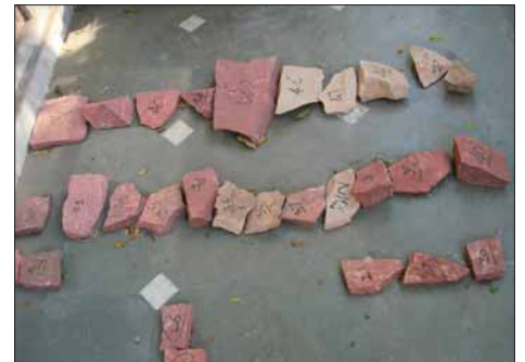
Almost 15% of sandstone on the neck of the dome is to be replaced
