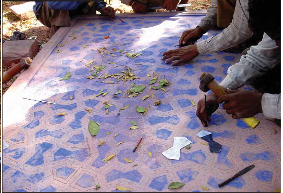
Carving of the traced jalli pattern
