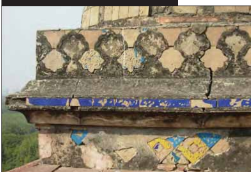
Original tilework on the canopies
