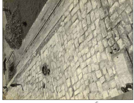
Archival pictures showing the lower plinth with the stone paving and the concrete being laid in 1956 to cover the paving, which, by then, had settled unequally
