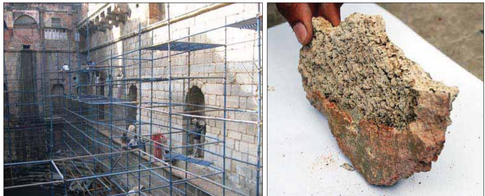
Removing epoxy layer and cement mortar
