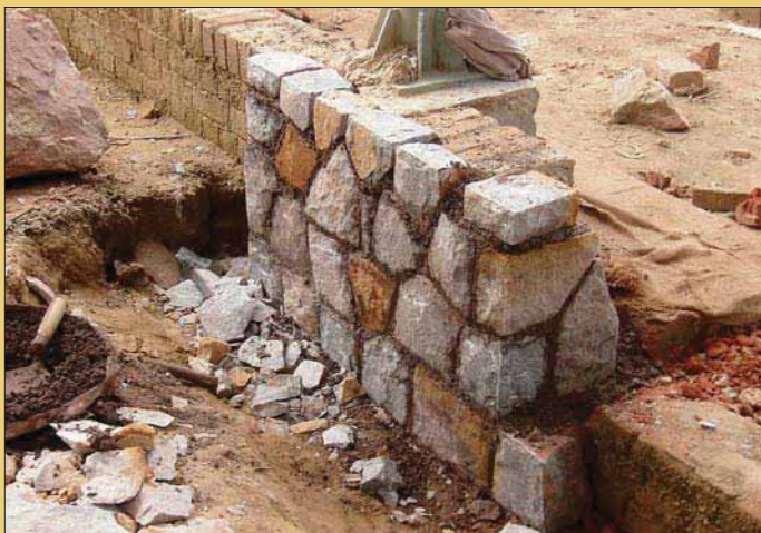
Cladding of Delhi Quartzite on the external walls
