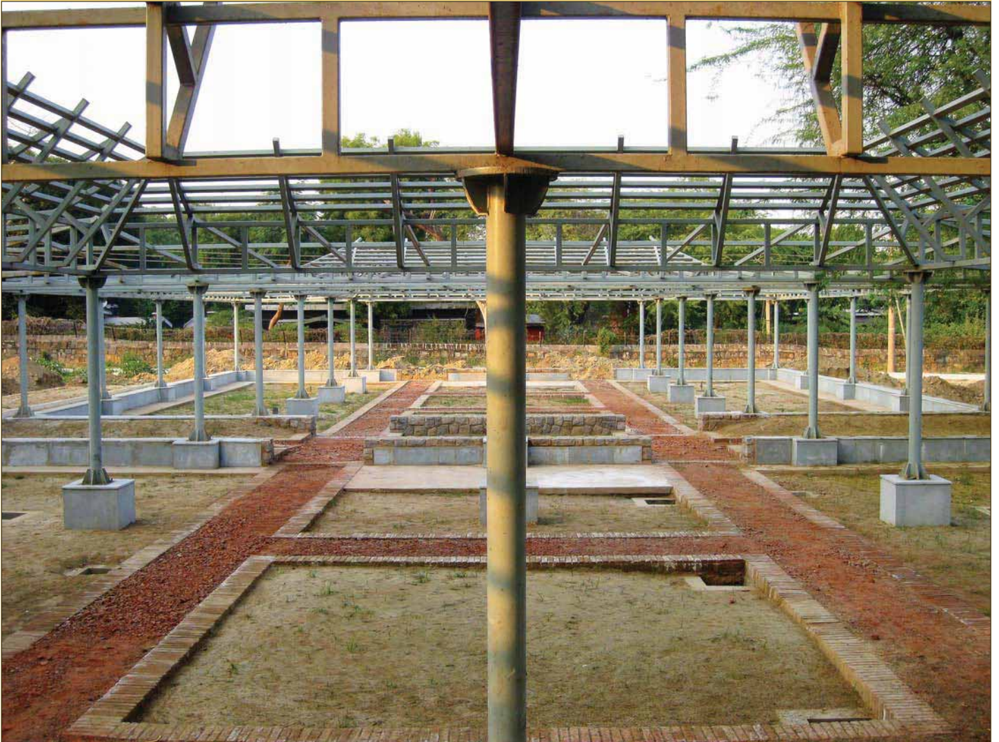
The elegantly designed nursery structures are now ready. An intricate lattice will soon roof the truss following which the structure is planned to host unique plant species.
