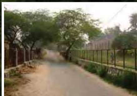
Shifting of Road
