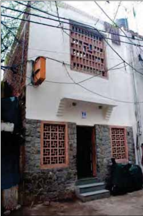
(Top) The construction and management of Community Toilet Complex in Nizamuddin Basti, adjacent to the Baoli gate of the Dargah, was completed in September 2009. It provides improved access to hygienic sanitation services to the residents of the Basti, a significant proportion of whom rely on public toilets.
