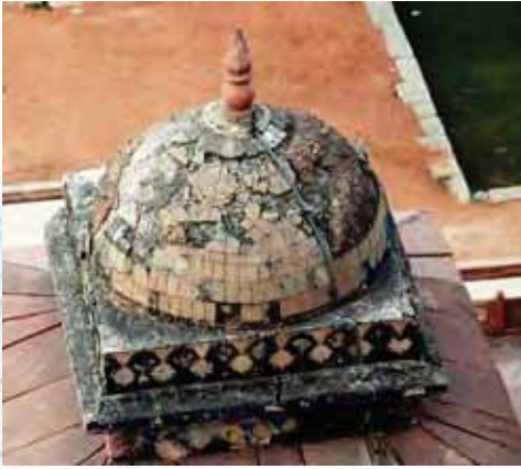
Condition mapping of the existing canopies on the roof
