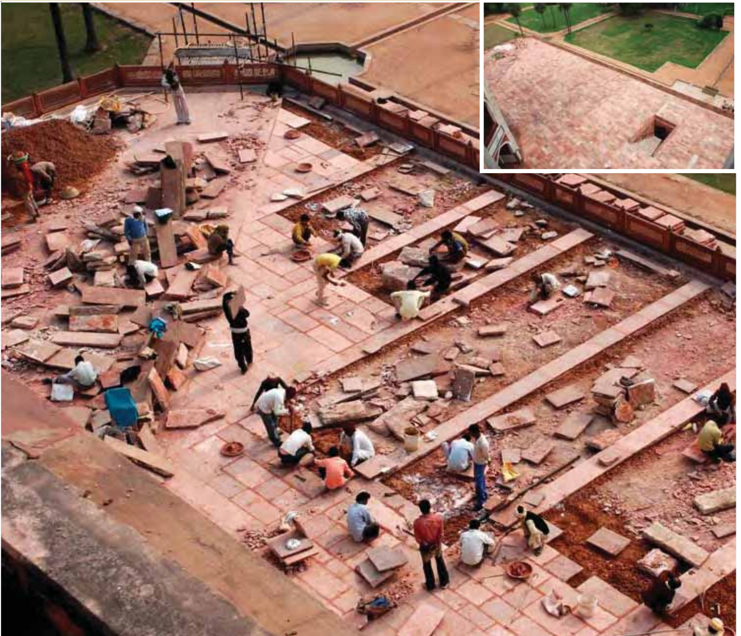
Re-Setting of Sandstone on the Upper Platform
