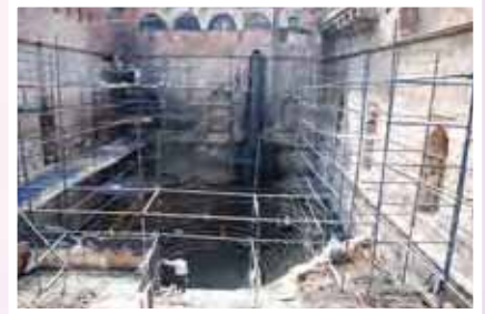
Conservation works in progress
