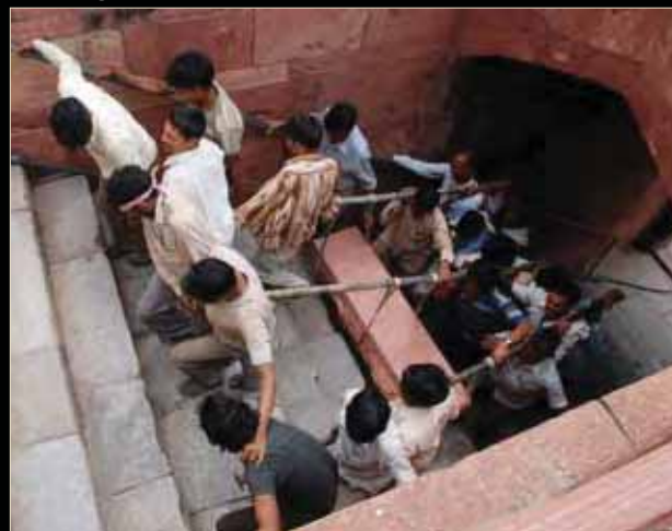
Re-Setting of Sandstone on the Upper Platform
