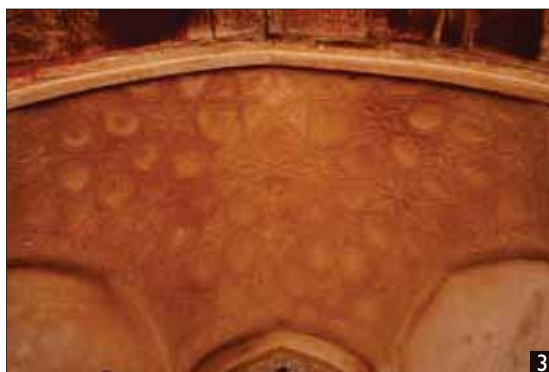
2 & 3. The restored pattern in lime mortar
