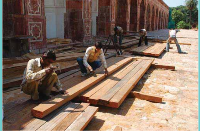
▲ Installation of wooden doors on 68 chambers, as per the original design
