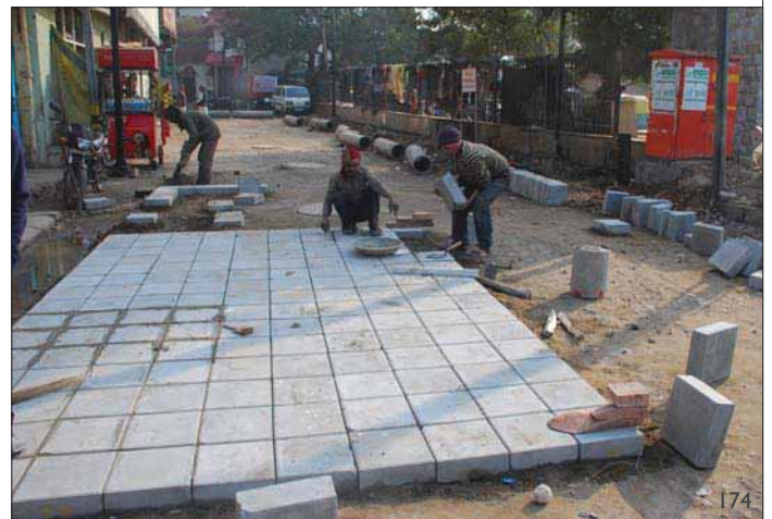
Street Improvement works underway ▼
