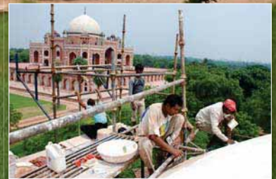
Protective lime plastering on the dome ▲
