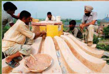
Craftsmen installing ceramic tiles on the finial of the Barber's Tomb ▲
