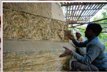
▲ Layers of soot required to be carefully cleaned using sandpaper
