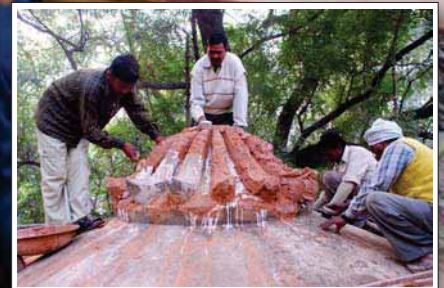
▲ The lotus motif on the lower finial required careful conservation to restore its original profile
