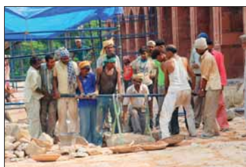
Stone paving of the lower plinth ▲
