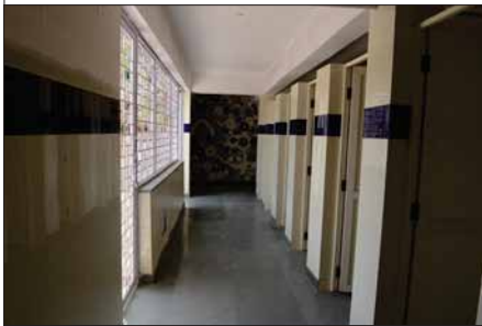
▲ View of the Toilet in 2008 ;View of the toilet complex in 2012
