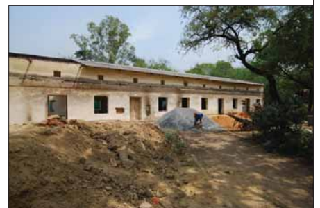
▲ A shed built in 1980's has been converted to serve as the project's site office
