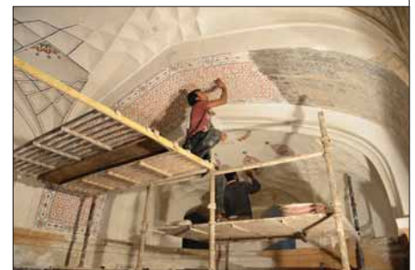
▲ Reconstruction of the missing incised plaster pattern on the dome ceiling, arch soffits and internal wall surfaces
