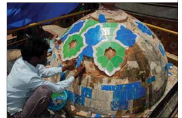
The restoration of the tile-work on the canopies on the roof ►
