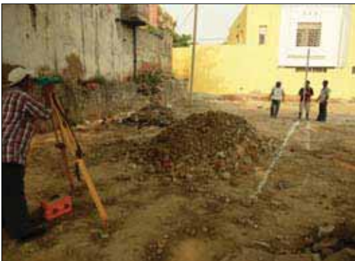
(Above) Initial survey and levelling works at Triangular Park
