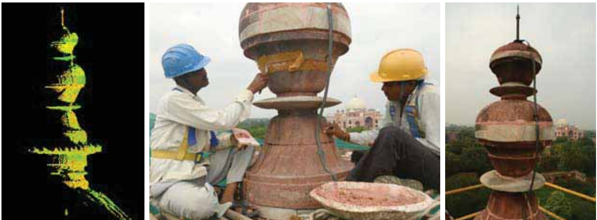
(Left) Finial of Nila Gumbad- Image generated using 3-D laser scanning Data (Centre) Craftsmen restoring the stone finial which is at the height (Right) Finial restored
