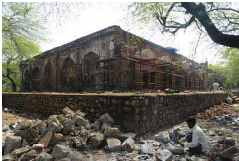
(Left) Consolidation of the collapsed portions and (Below) View of South facade of Mirza Muzaffar Hussain's Tomb during conservation
