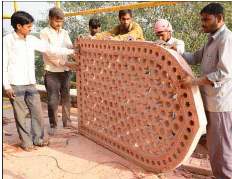
(Left) The craftsmen transporting the sandstone jaali weighing over 700kg to the height of over 40 feet (Right) It takes 2-3 months of hardwork by 8 craftsmen to prepare a jaali of this size and complexity. All the 8 sandstone lattice screens on the neck of the dome and 4 lattice screens on the lower level are restored.
