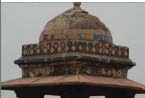
(Below) Various stages of tile restoration on the canopies
