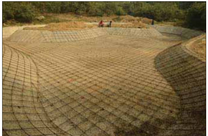
(Left) Layout and marking of rivulets on site; (Right) Construction of Concrete Beds
