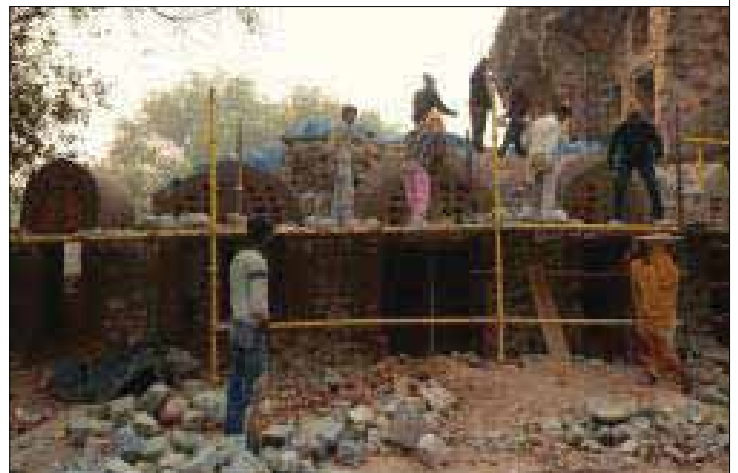
(Left) Image showing collapsed vaulted chambers (Right) Vaulted Chambers after the conservation works
