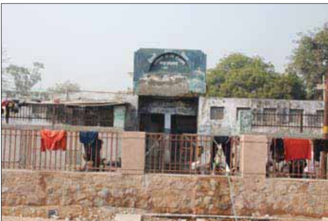
Community Toilet Complex in 2009
