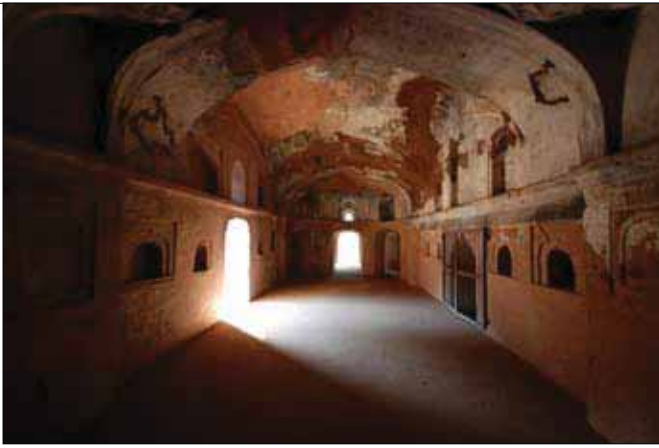
(Above) Before & After Conservation views of the internal chambers of Mirza Muzaffar Hussain's Tomb after the restoration of missing geometric patterns in incised plasterwork on the interior wall and roof surfaces
