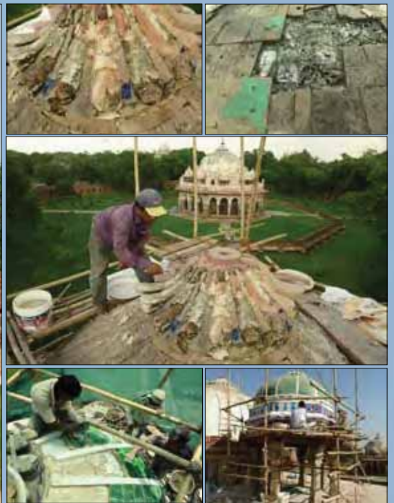
(Left) Isa Khan's Mosque in 2011, before conservation; (Right) Various stages of tilework restoration on canopies and finial
