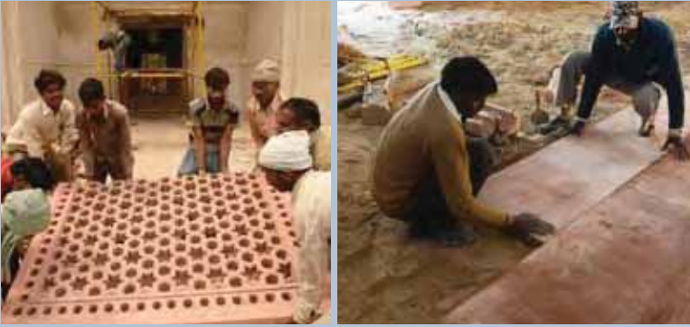
Reinstalling Sandstone jaalis and paving
