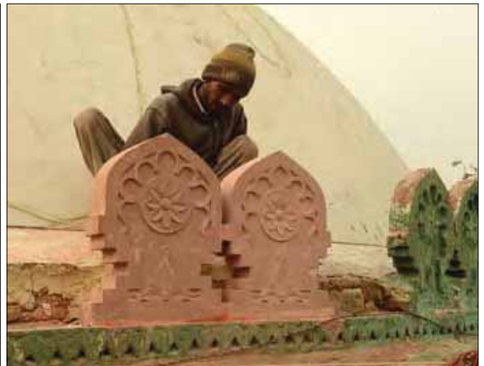
Conservation works at the 14 th century Khilji mosque required scrapping of several dozen paint and cement layers prior to repair or replacement of the damaged sandstone elements.
