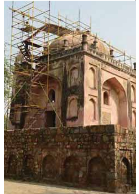
At the Mughal Tomb, a sandstone plinth replaced the earlier cement plinth (Below) which was found to have been laid over construction rubble. The sandstone is long lasting, especially in view of the large number of visitors expected to visit here in future years.
