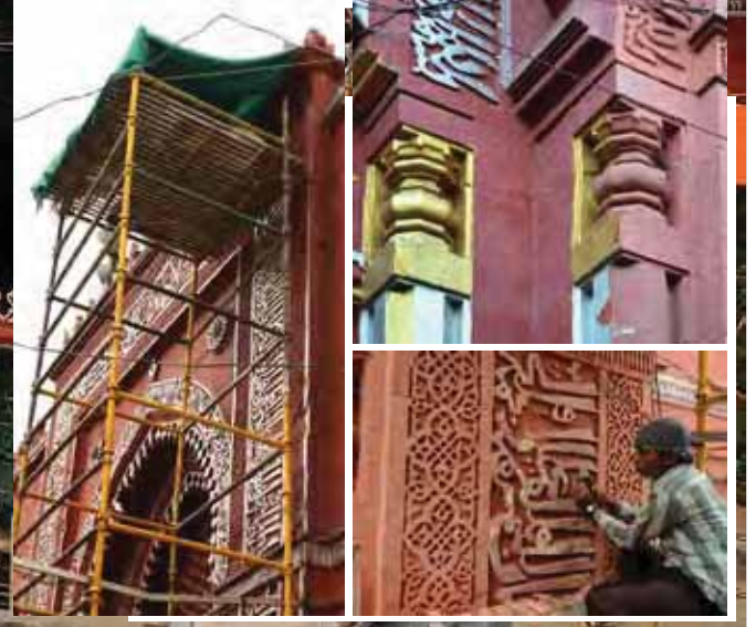
FACADE: During Conservation
