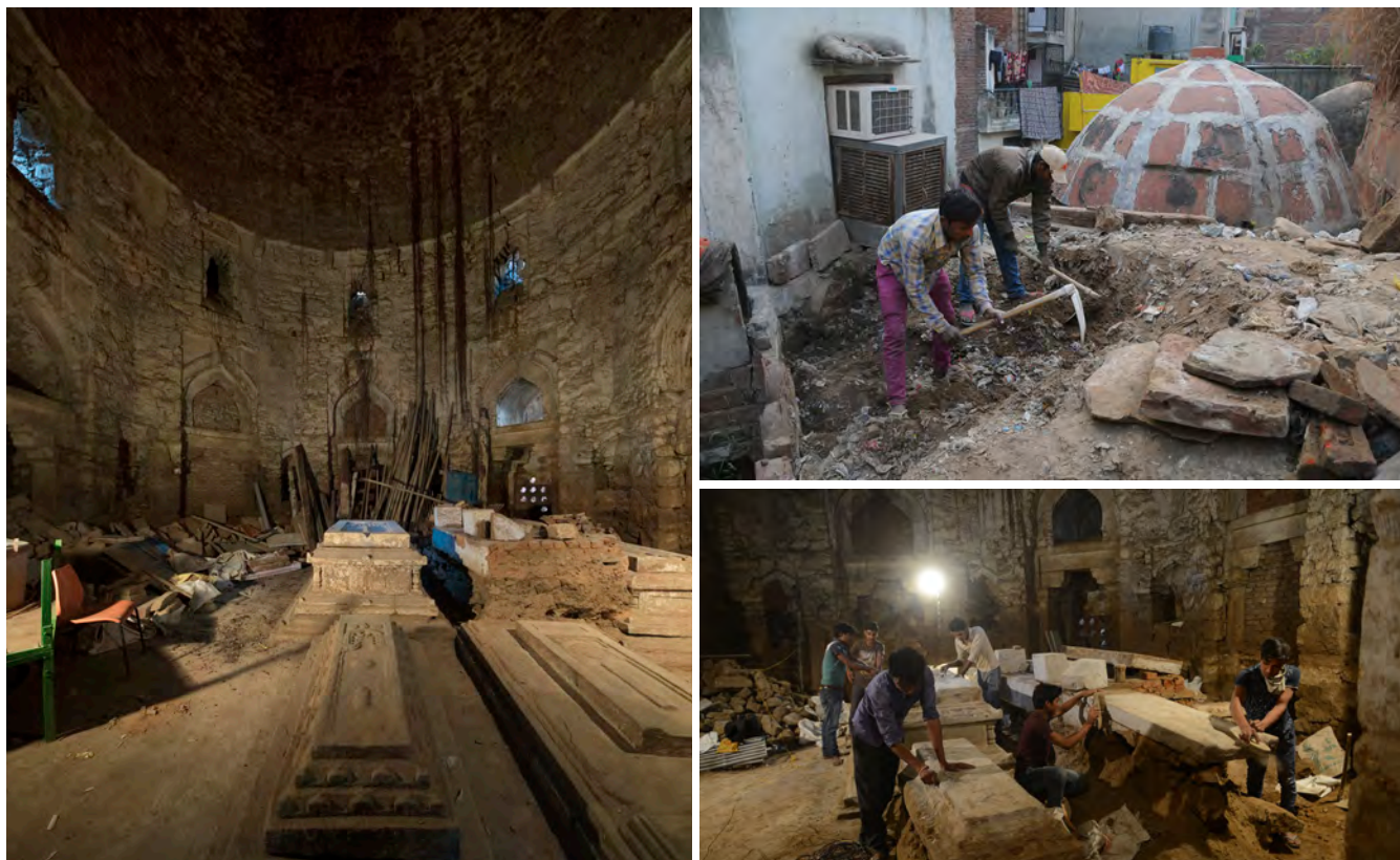
Removal of unplanned 20th century modern structures from the south facade.
