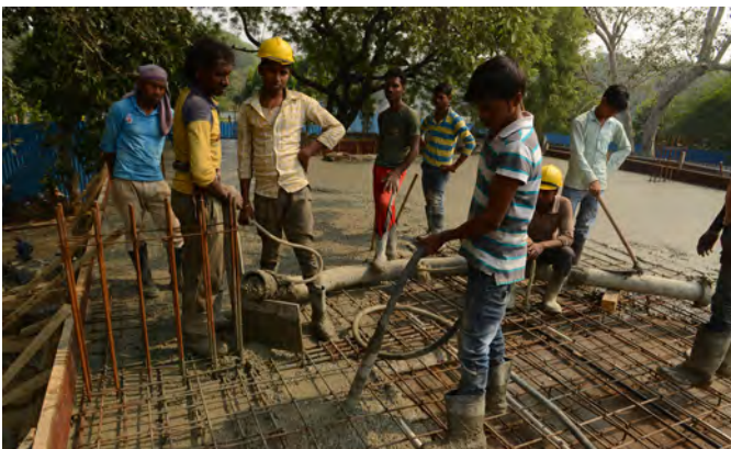
(Top) Interior View of principal gallery of Humayun's Tomb site museum; (Middle) Concreting process at the floor of administrative block of HTIC; (Bottom) Curing process of columns of administrative block
