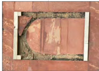
DETAIL OF RED SANDSTONE AND WHITE MARBLE ARCHES IN FACADE
