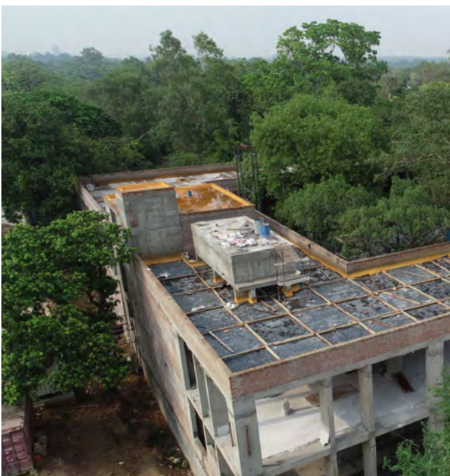
Dismantling of terrazzo flooring of North Chamber
