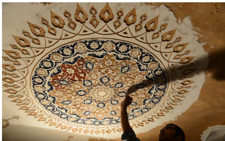
Ongoing conservation work on the ceiling of Mirza Muzaffar Hussain Mausoleum
