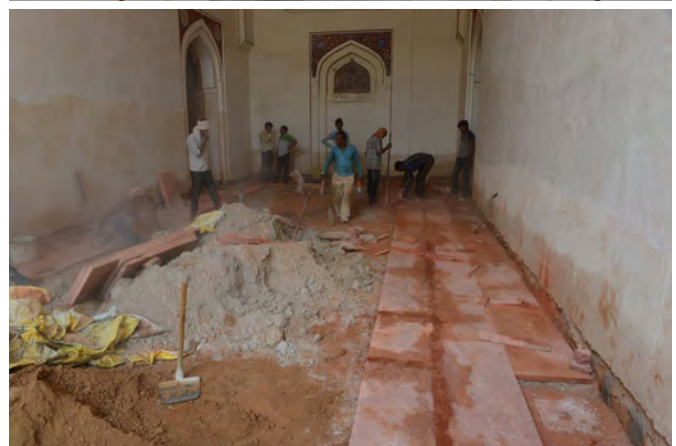
Clockwise from Top: Image of the medallion on ceiling; before and after images of arches restored with traditional paint; Dismantling of terazzo flooring; Layering of red sandstone flooring
