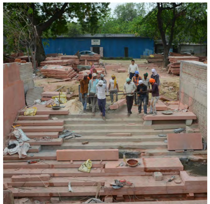
Laying of monolithic red sandstone blocks on the exit staircase towards Humayun's Tomb.
