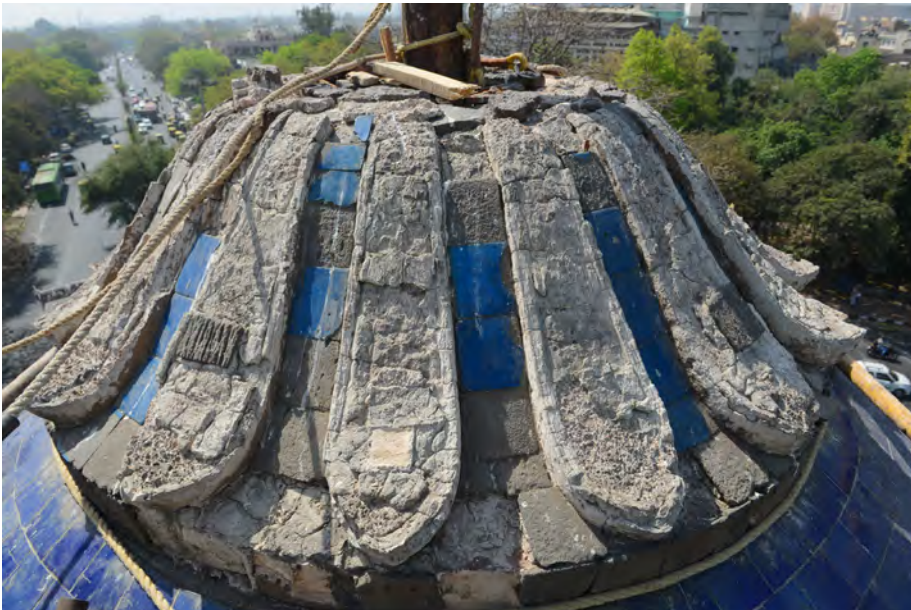
Missing tile work on the finial of the dome being restored with tiles matching the original
