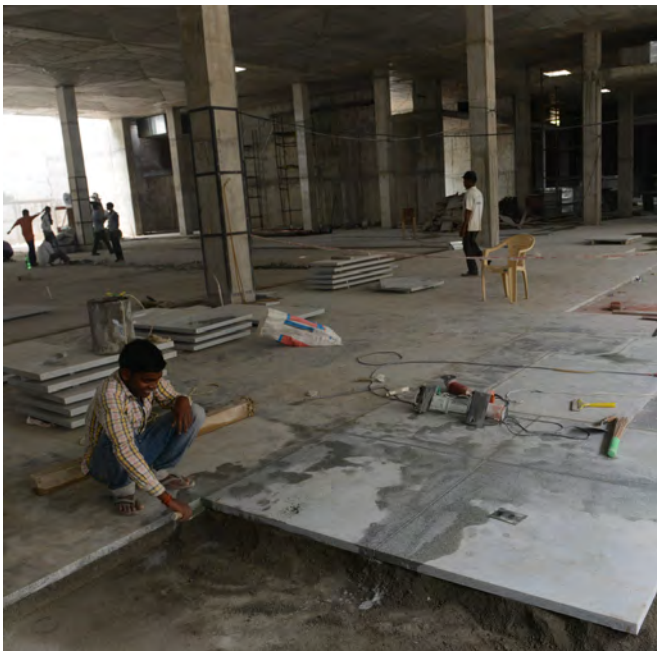
Laying of 40mm thick sadar-ali granite stone in main exhibition gallery.
