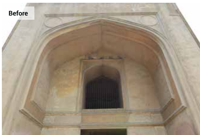
Conservation of one of the four principal facades. Note that the sandstone jaali's was restored as were the intricate incised plaster patterns.
