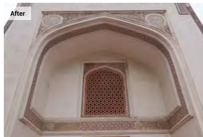
Conservation of one of the four principal facades. Note that the sandstone jaali's was restored as were the intricate incised plaster patterns.
