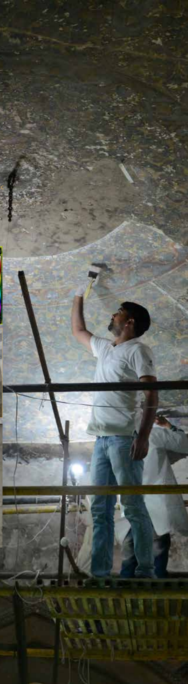
Thermal imaging revealed areas of dampness leading to loss of paint layers
