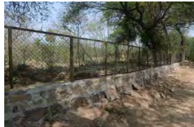
(Above) Newly constructed toilet near the lakeside (Below): boundary wall to safeguard habitat zone.
