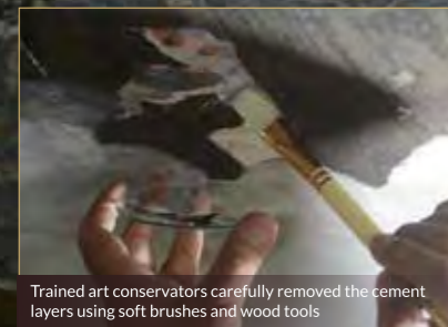
A thin layer of cement render covered the painted ceiling
