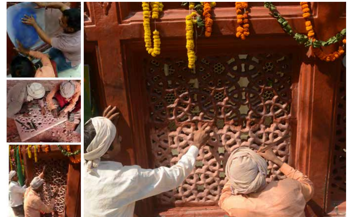
Repairs to the damaged jaali screens were carried out by master craftsmen
