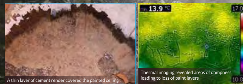
A thin layer of cement render covered the painted ceiling
