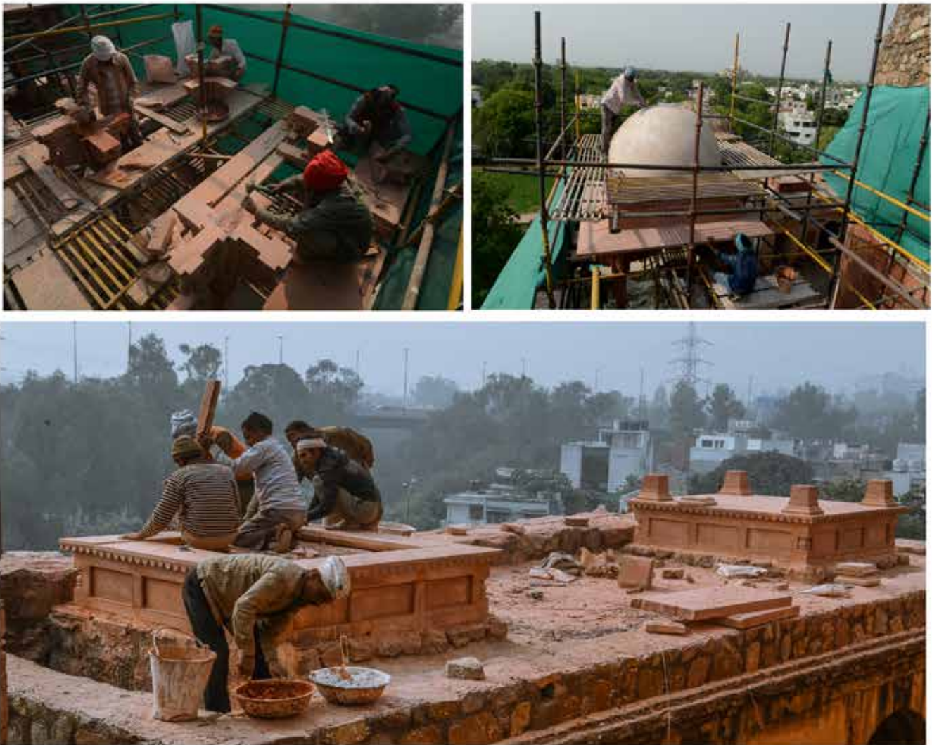
(Above) stone elements found at the site have been used to reconstruct four of the seven missing canopies
