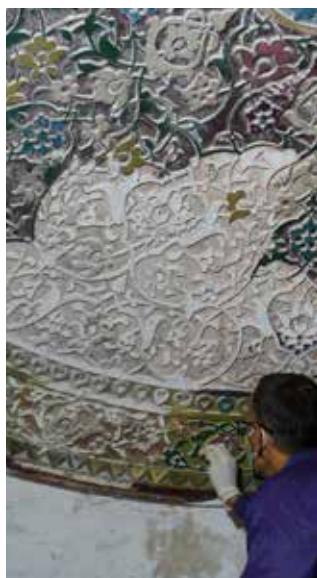
(Above) Craftsmen carefully removing layers of paint from the ceiling.
