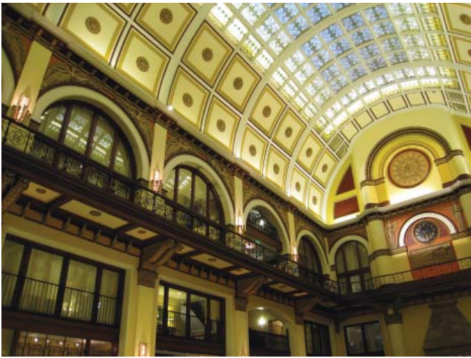
Fig. 1. A decorative, stained glass skylight allows natural daylight into the interior.
