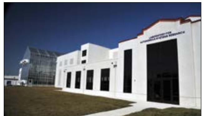
This facility on the Washington, D.C., campus is a nerve center for basic research in autonomous systems for the Navy and Marine Corps.
