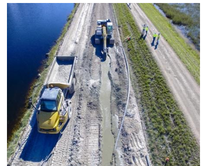
Deep Soil Mixing
