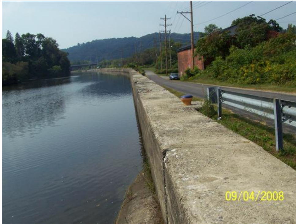
Figure 6-7: Concrete Wall along Canal at Little Falls, NY
