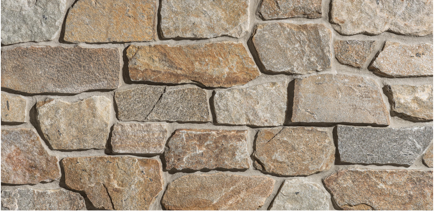
Photo Shows Installation With Mortar Joint
