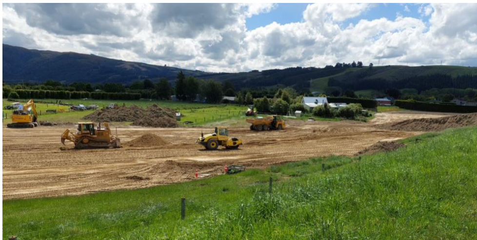
Figure 8: Construction progressing at Outram site (22 November 2022).
