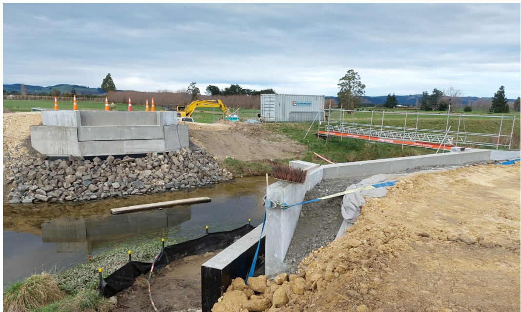
Figure 7: Bridge 11 replacement underway at Contour Channel (18 July 2023).
