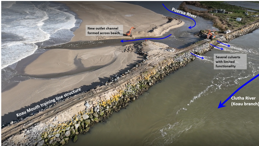
Figure 21: The coastline impact of the Puerua Estuary and Lower Clutha Flood Protection and Drainage Scheme infrastructure (5 July 2023).
