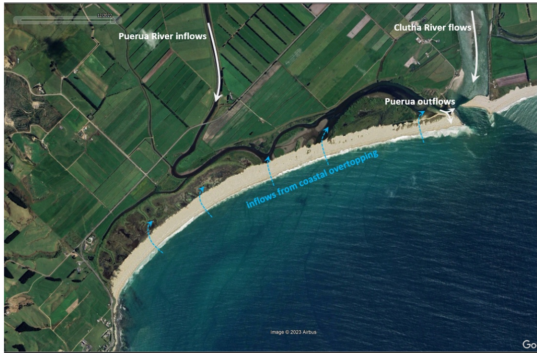
Figure 18: River outflows and coastal overtopping at the Puerua River estuary.
