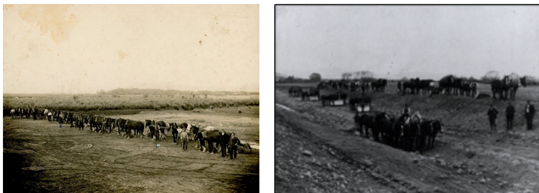
Figure 4 and 5: Contour Channel construction early 1900's.
