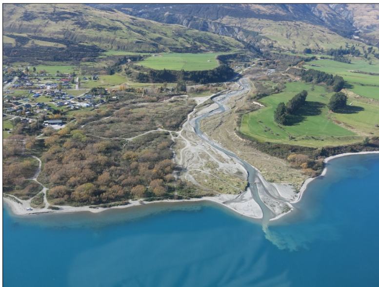
Figure 2: Overview of the Buckler Burn stream and alluvial fan, with Glenorchy township located the northern side of stream's active channel. The full township area is developed on Buckler Burn alluvial fan deposits, and the higher terraces to each side of the stream are remnants of older alluvial fan-delta surfaces formed when the lake was at higher levels. Photograph dated May 2018.
