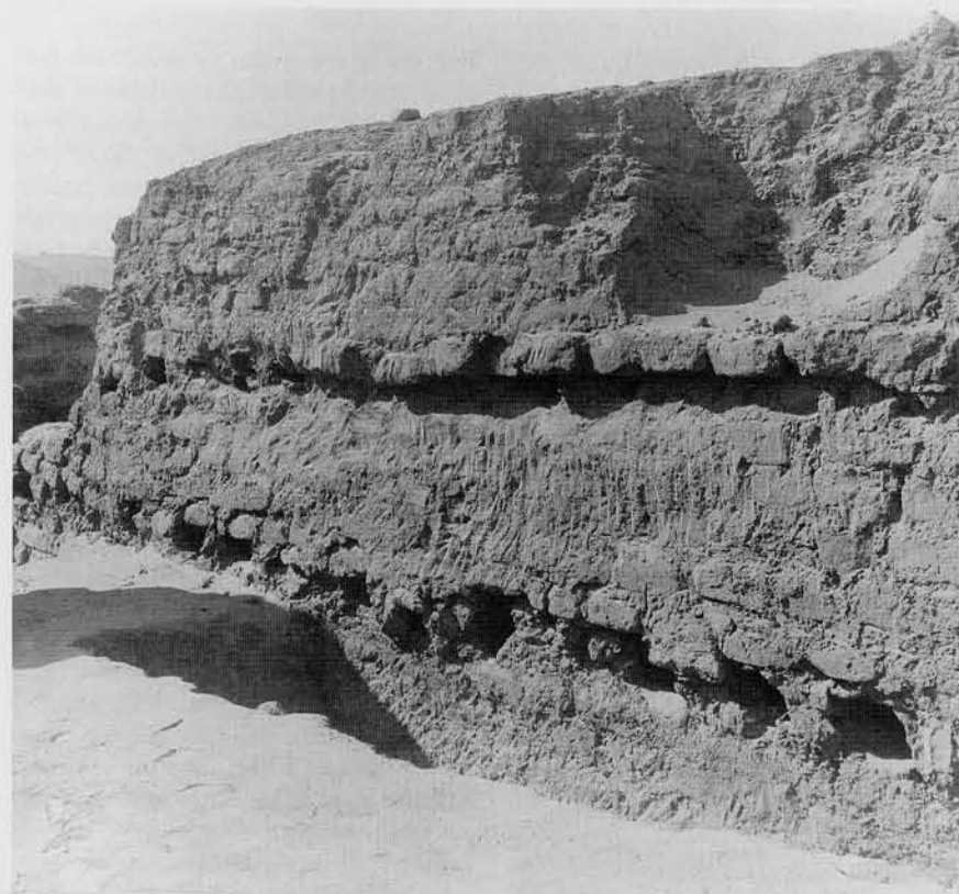
5 The mud brick walls of the square building at Tell el-Kheleifeh were pierced by two rows of holes. These holes, originally interpreted by Glueck as part of an elaborate system of flues for a giant refining installation, are more likely the remnants of wooden beams placed to protect the walls from earthquake damage. (From the ASOR collection at the Harvard Semitic Museum)
