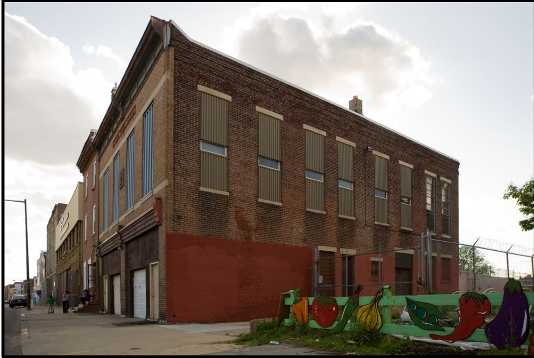
Figure 6. Top: Looking west at the primary (southeast) and side (northeast) elevations. Source: Brad Maule, 2014.
