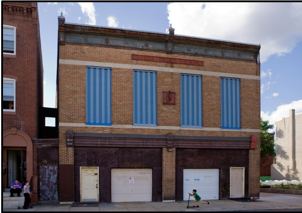
Figure 1. The primary (southeast) elevation. Source: Brad Maule, 2014.
