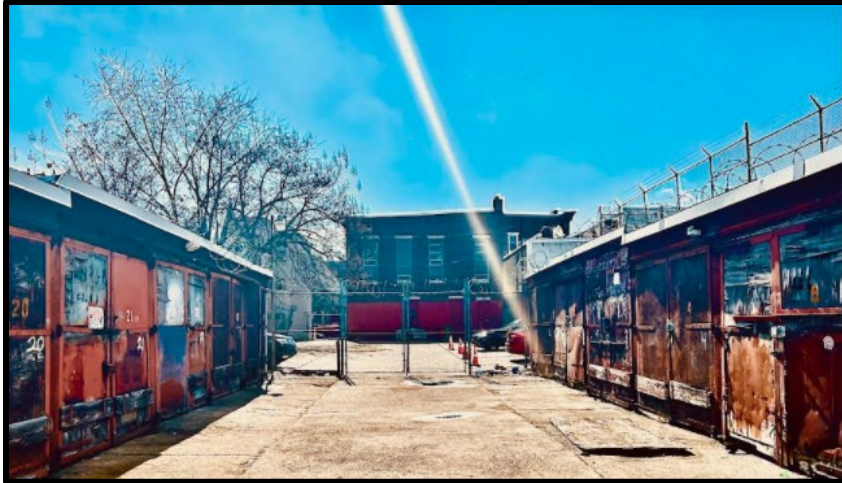
Figure 7. Top: The entrance of the Ioska Tribe at the rear of the Side (Northeast) Elevation. Figure 8. Bottom: Looking southeast at the Rear (Northwest) Elevation of the subject building through a court of garages built to subsidize the fraternal organization in the 1920s. Source: Oscar Beisert, 2022.
