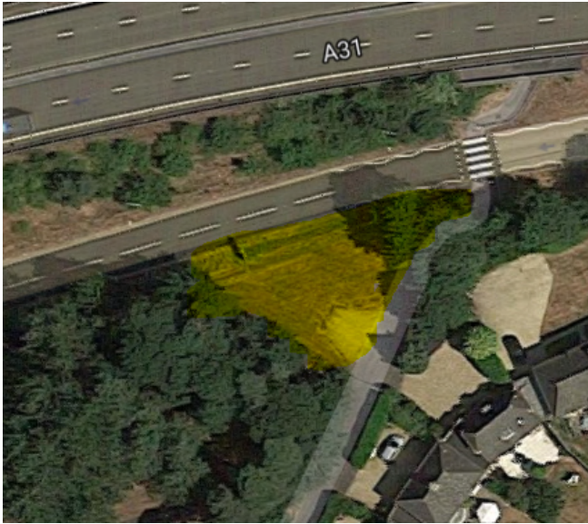
1 – Underpass leading to Linden Gardens
