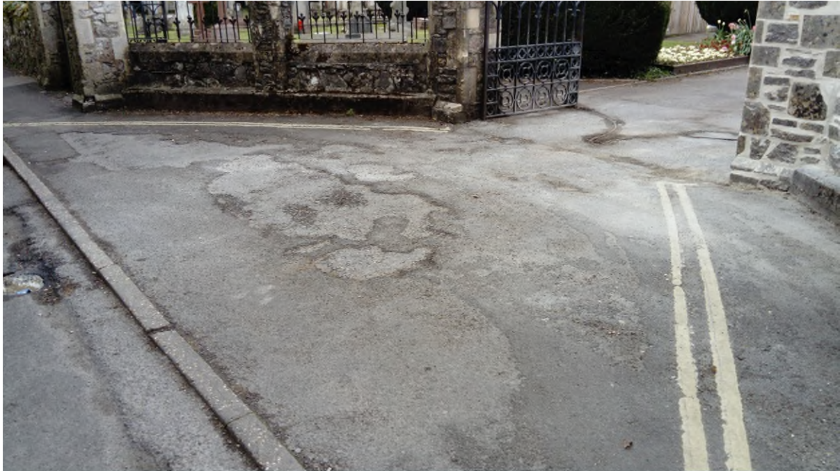
Figure 1 - Tarmac surface at entrance
