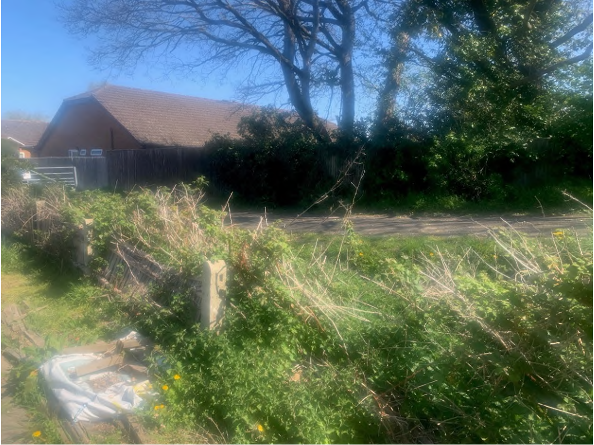
Figure 1 – Dilapidated and overgrown fence at entrance to allotments site
